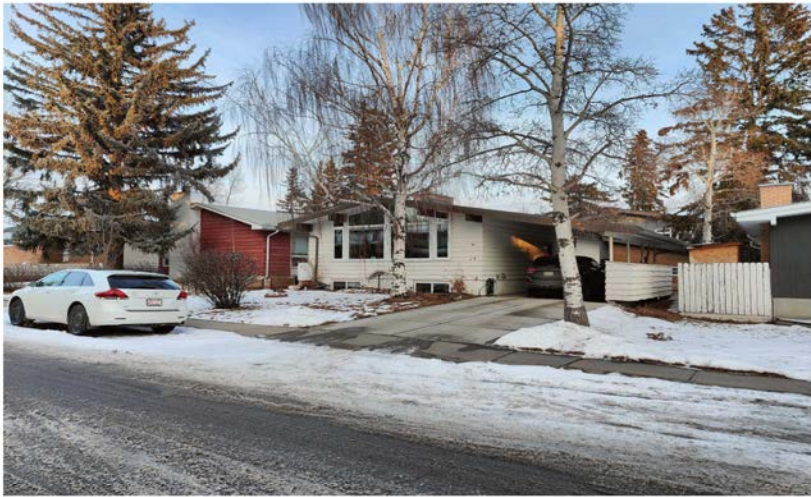
1 FRONT VIEW - NORTH NEIGHBOUR - 28 GISSING DR. SW
