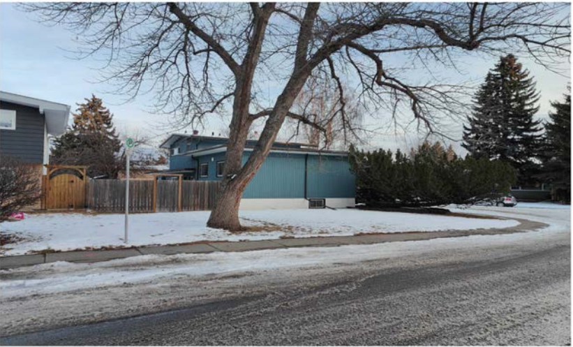
3 FRONT VIEW - SOUTH NEIGHBOUR - 20 GISSING DR. SW
