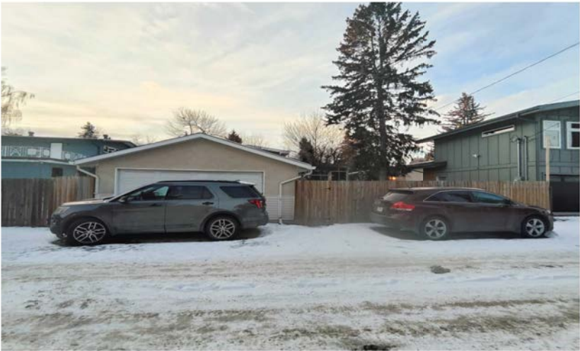
6 REAR VIEW - SUBJECT PROPERTY - 24 GISSING DR. SW
