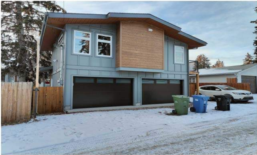
5 REAR VIEW - NORTH NEIGHBOUR - 28 GISSING DR. SW
