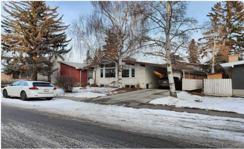
1 FRONT VIEW - NORTH NEIGHBOUR - 28 GISSING DR. SW
