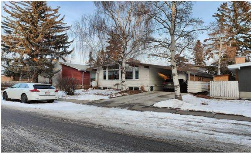
1 FRONT VIEW - NORTH NEIGHBOUR - 28 GISSING DR. SW
