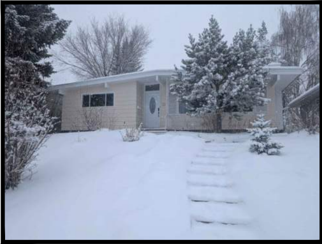
F EAST OF NORTH "FRONT" ELEVATION VIEW WEST OF NORTH OF VIRGINIA DRIVE NW LOOKING WEST
