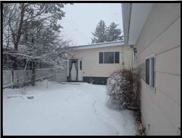
K SOUTH REAR YARD VIEW SOUTH OF REAR YARD LOOKING NORTH
