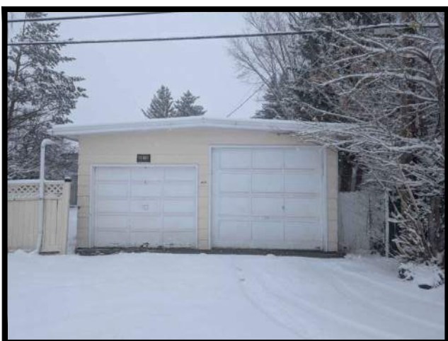
O SOUTH REAR ELEVATION VIEW SOUTH OF REAR LANE LOOKING NORTH
