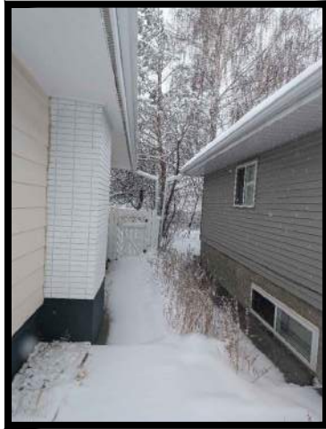
G WEST "RIGHT" SIDE YARD VIEW WEST OF PROPERTY WEST OF SOUTH
