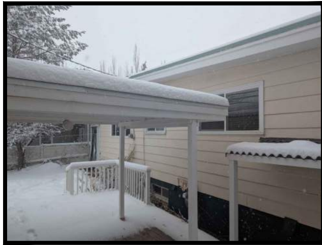
L EAST REAR YARD VIEW EAST OF PROPERTY LOOKING WEST
