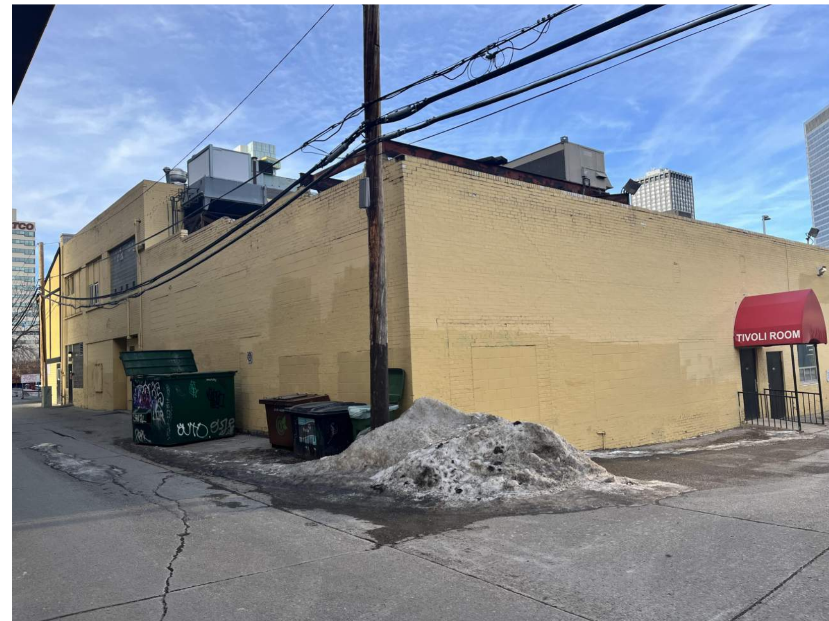
2. SOUTHEAST CORNER VIEW
