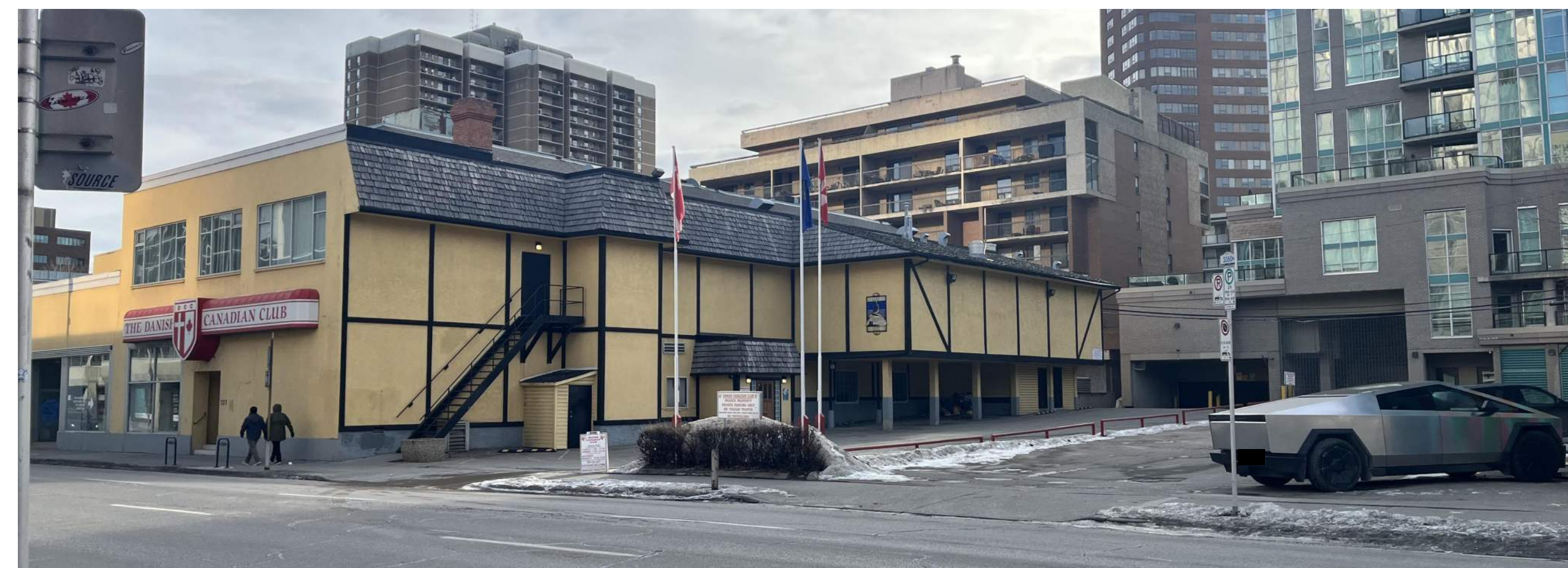
4. NORTHWEST CORNER VIEW
