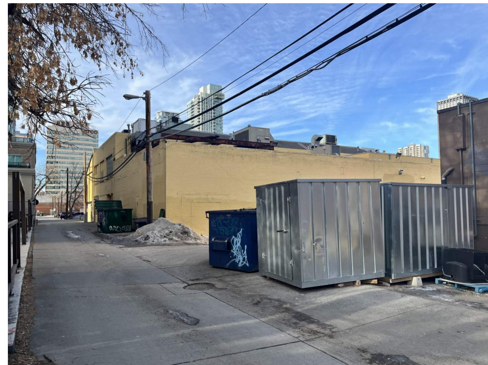
2. SOUTHEAST CORNER VIEW
