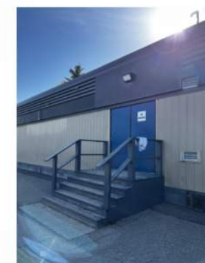
PHOTO 7. NEW MODULAR LOCATION
