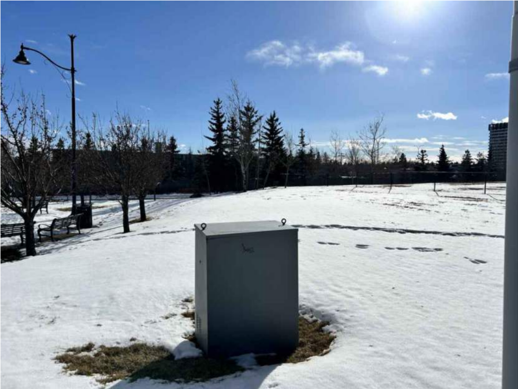
1.0 - Looking South West
