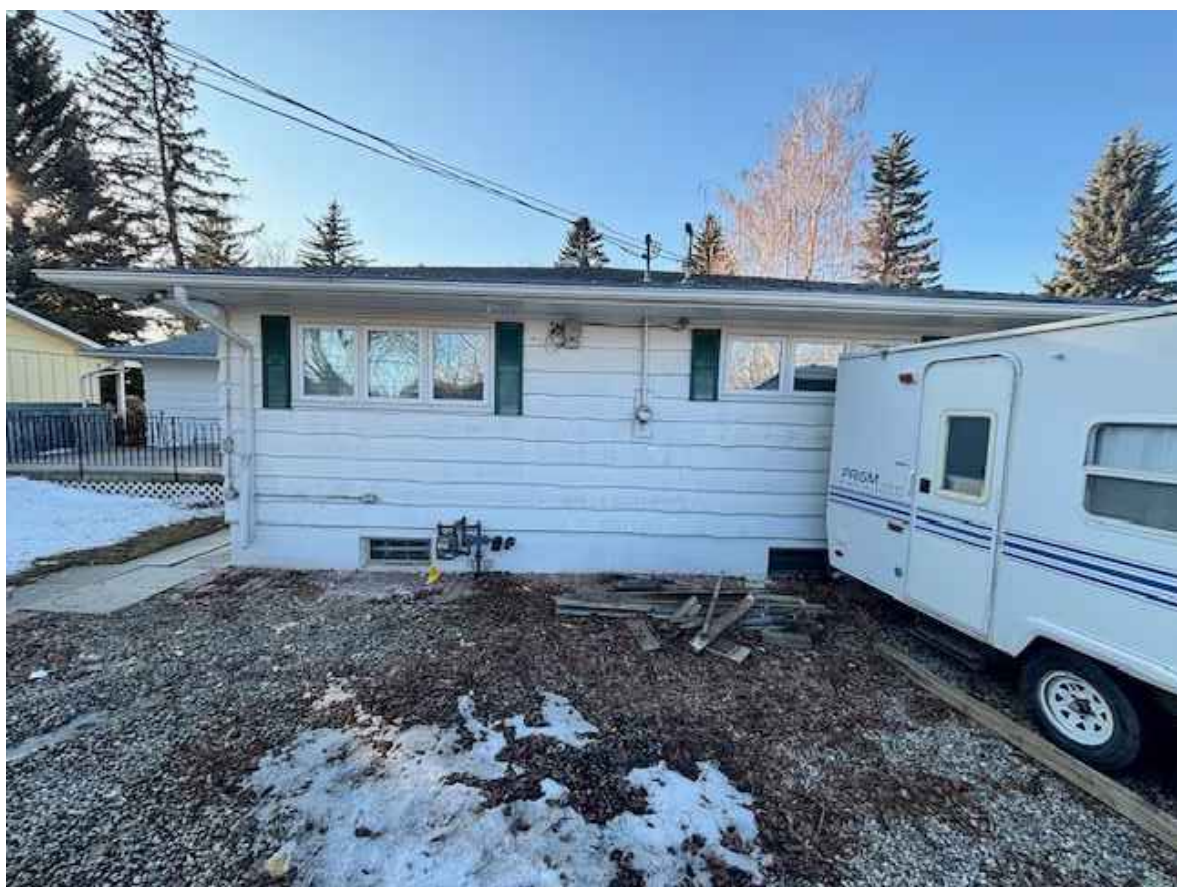
6 SITE PHOTO DP1.2 SCALE: NTS
