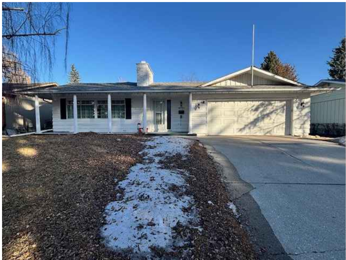
2 SITE PHOTO DP1.2 SCALE: NTS
