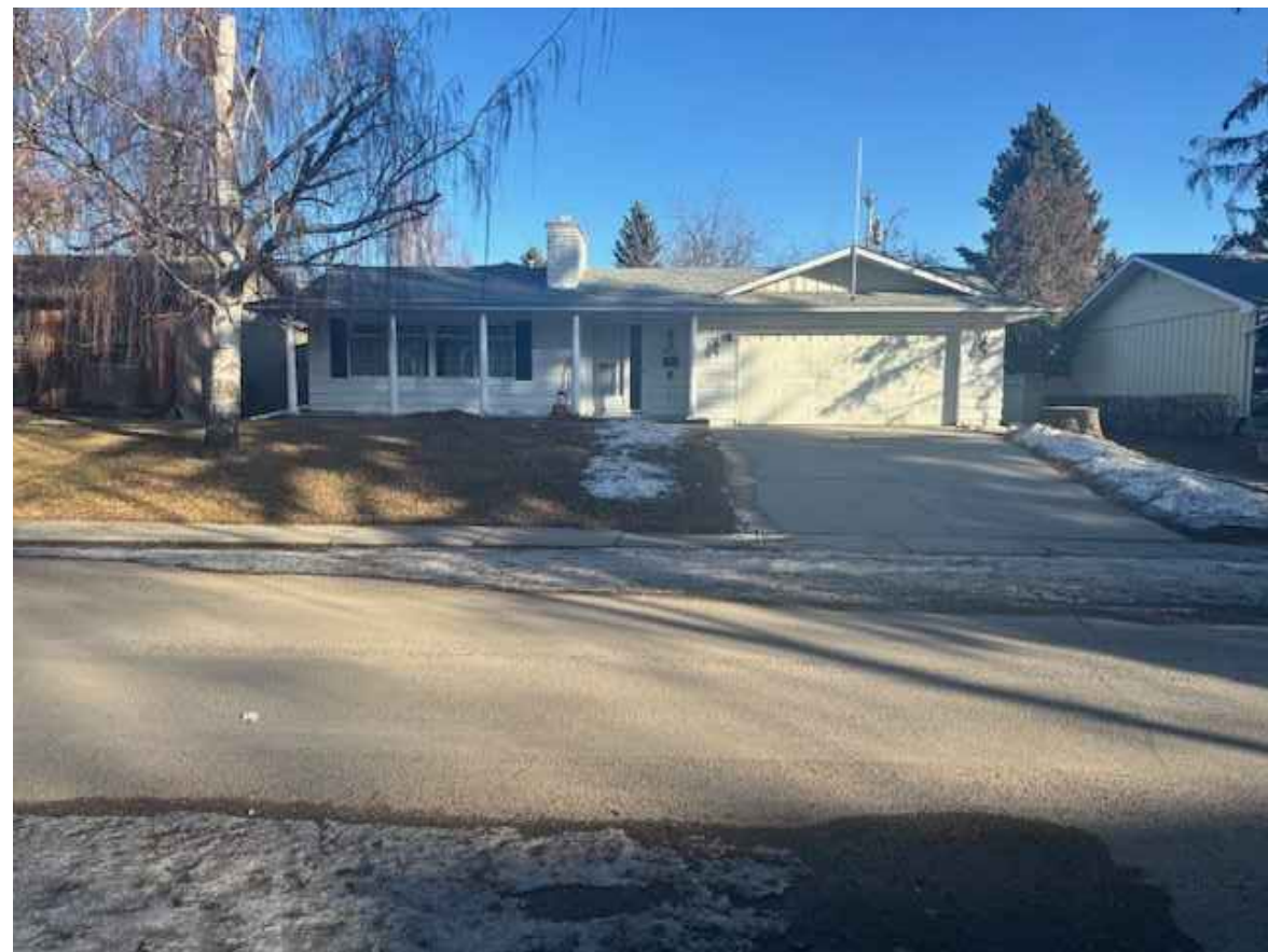
1 SITE PHOTO DP1.2 SCALE: NTS
