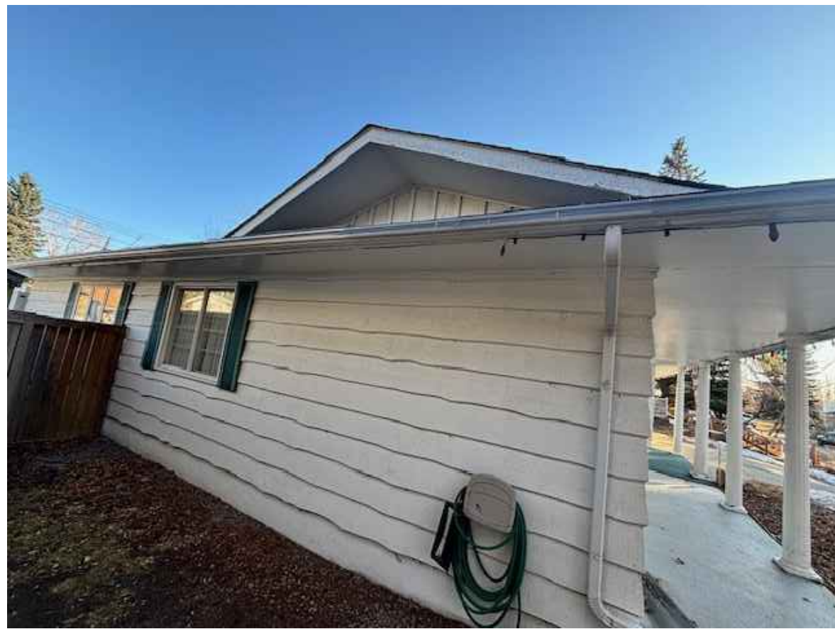
7 SITE PHOTO DP1.2 SCALE: NTS
