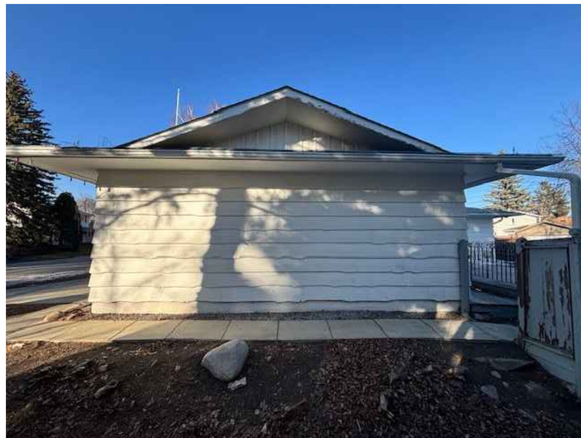
3 SITE PHOTO DP1.2 SCALE: NTS
