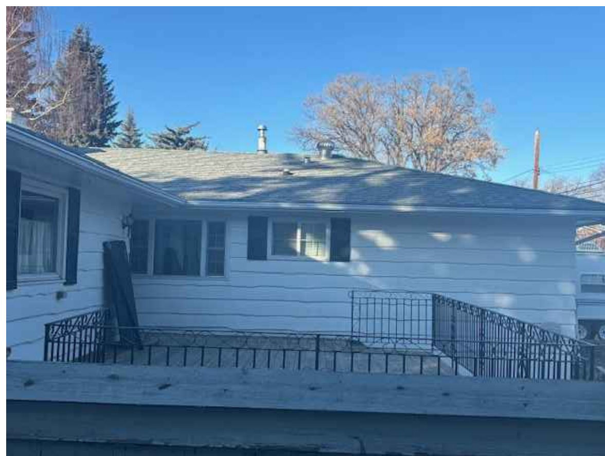
5 SITE PHOTO DP1.2 SCALE: NTS
