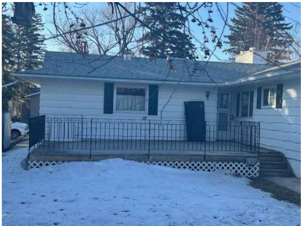
4 SITE PHOTO DP1.2 SCALE: NTS
