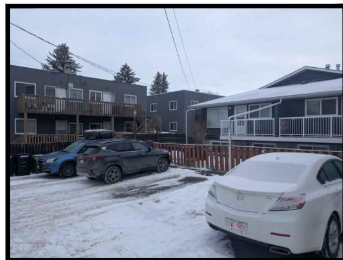
I | SOUTHWEST 'REAR YARD' VIEW SOUTHWEST OF PROPERTY LOOKING NORTHEAST
