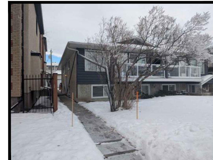
M | SOUTHEAST 'FRONT ELEVATION' VIEW SOUTHEAST OF PROPERTY LOOKING NORTHEAST
