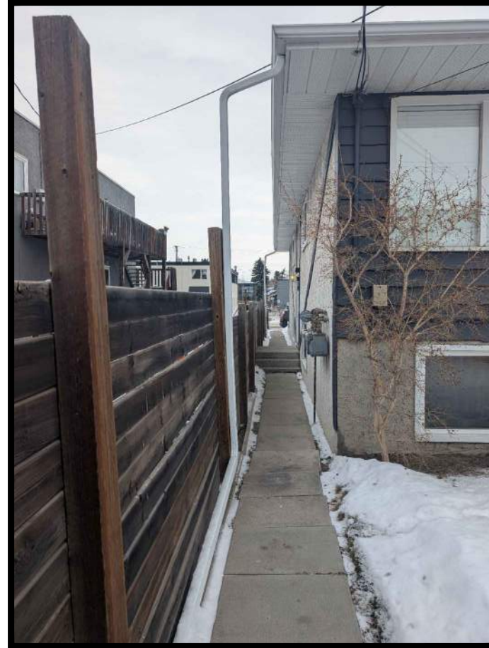
E | NORTH 'RIGHT SIDE YARD' VIEW NORTH SIDE OF PROPERTY LOOKING EAST
