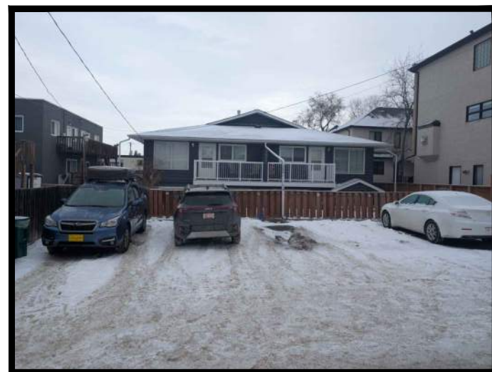
J | WEST 'REAR YARD' VIEW WEST OF PROPERTY LOOKING EAST
