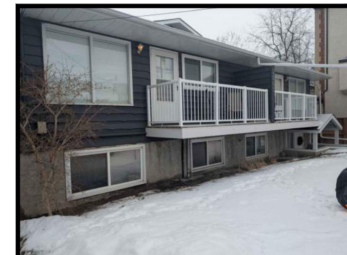
L | NORTH 'REAR ELEVATION' VIEW NORTH SIDE OF PROPERTY LOOKING SOUTH
