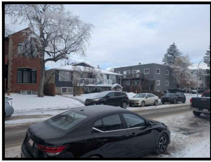
A | EAST "STREETSCAPE" VIEW SOUTHEAST OF 14A STREET SW LOOKING NORTHWEST
