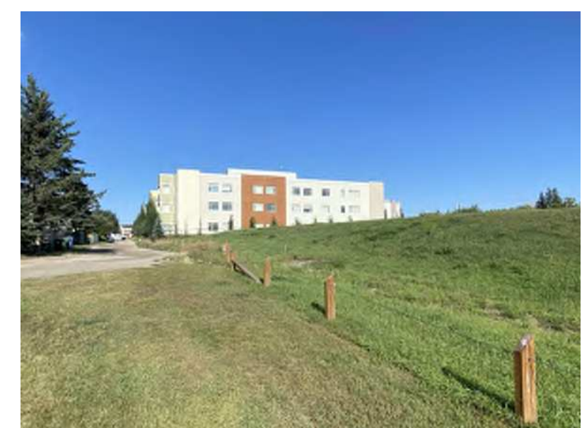
SITE PHOTO - VIEW FROM SE LOOKING TO WEST EDGE OF SITE AND ADJACENT BUILDING
