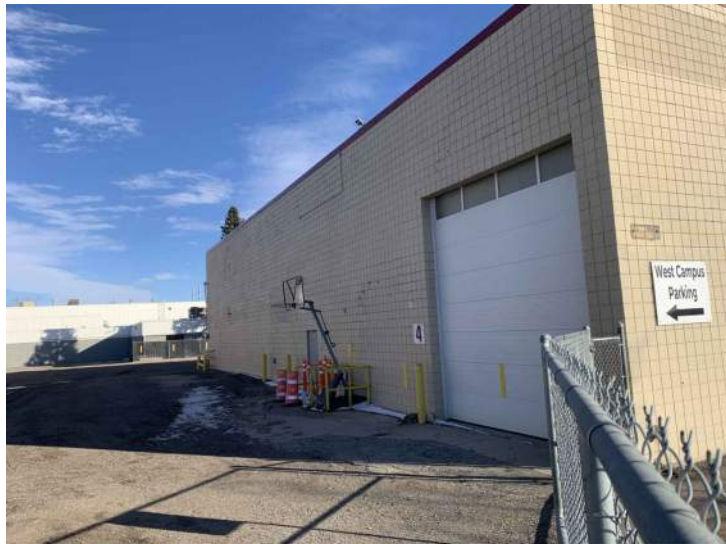
VIEW OF NORTH ELEVATION
