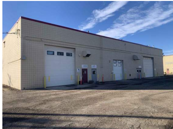
VIEW OF EAST ELEVATION
