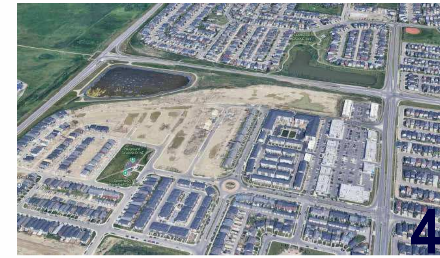
AERIAL VIEW WEST
