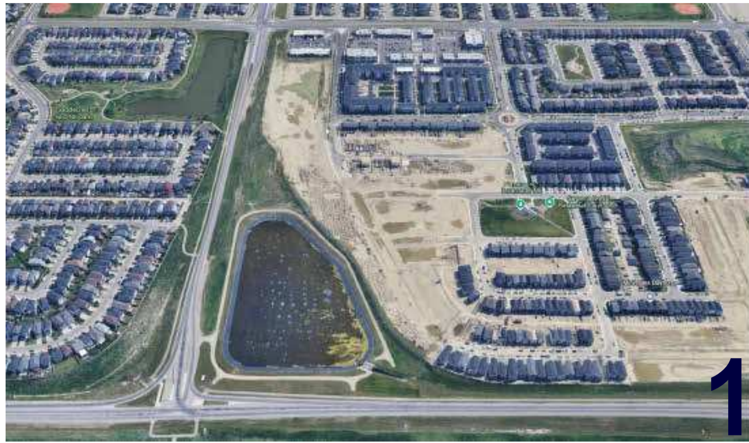
AERIAL VIEW NORTH
