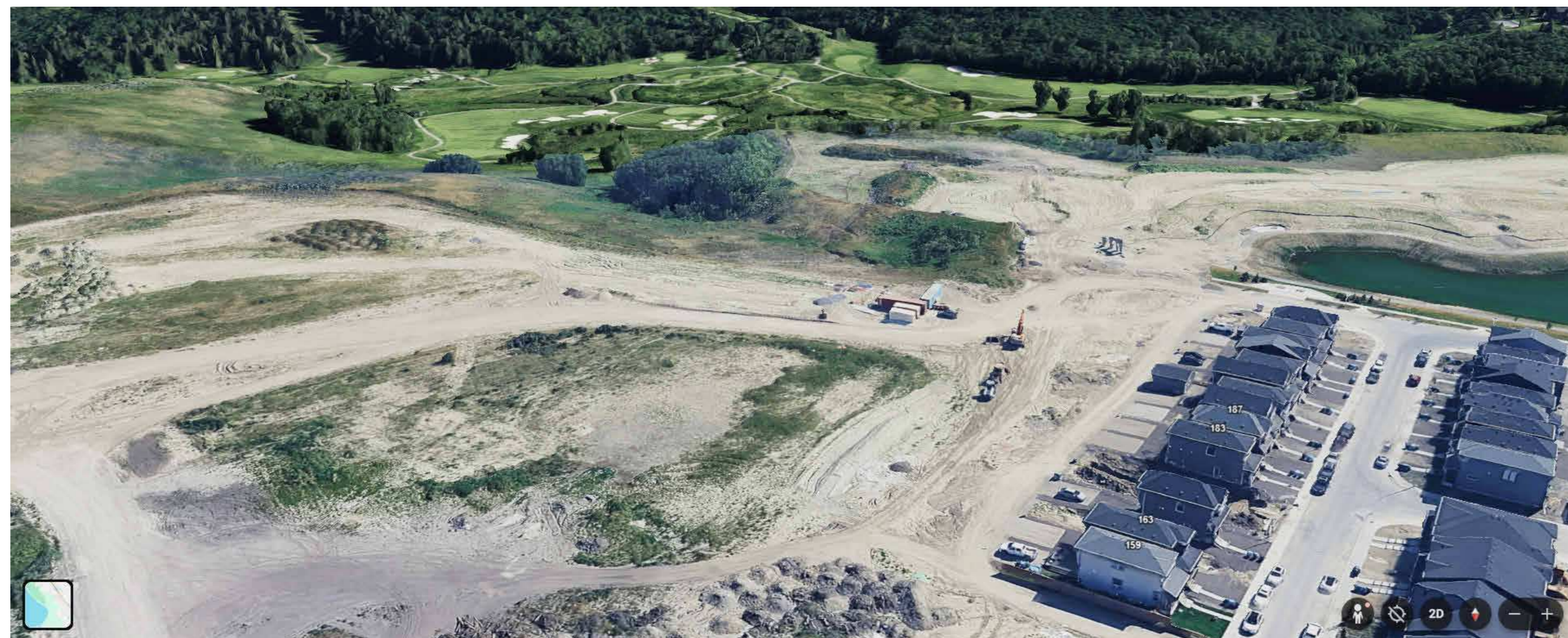
SITE PHOTO - SOUTH
