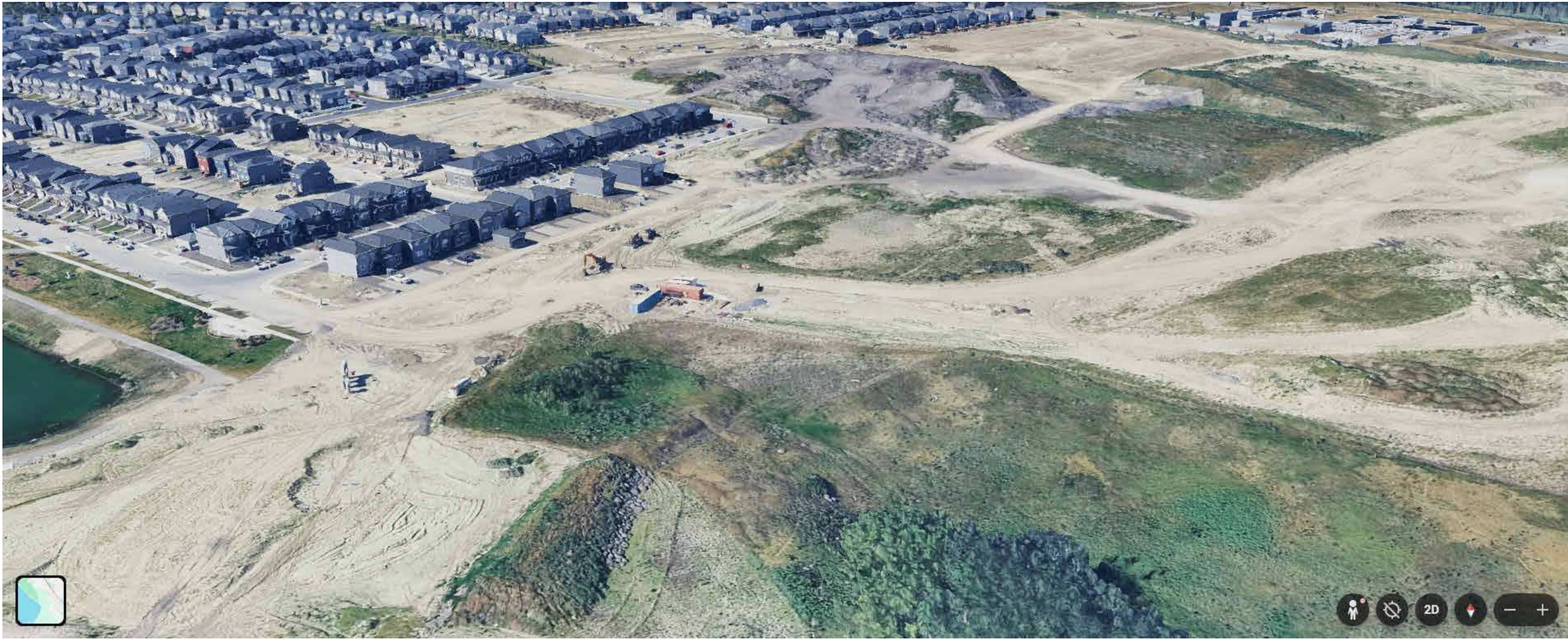
SITE PHOTO - NORTH
