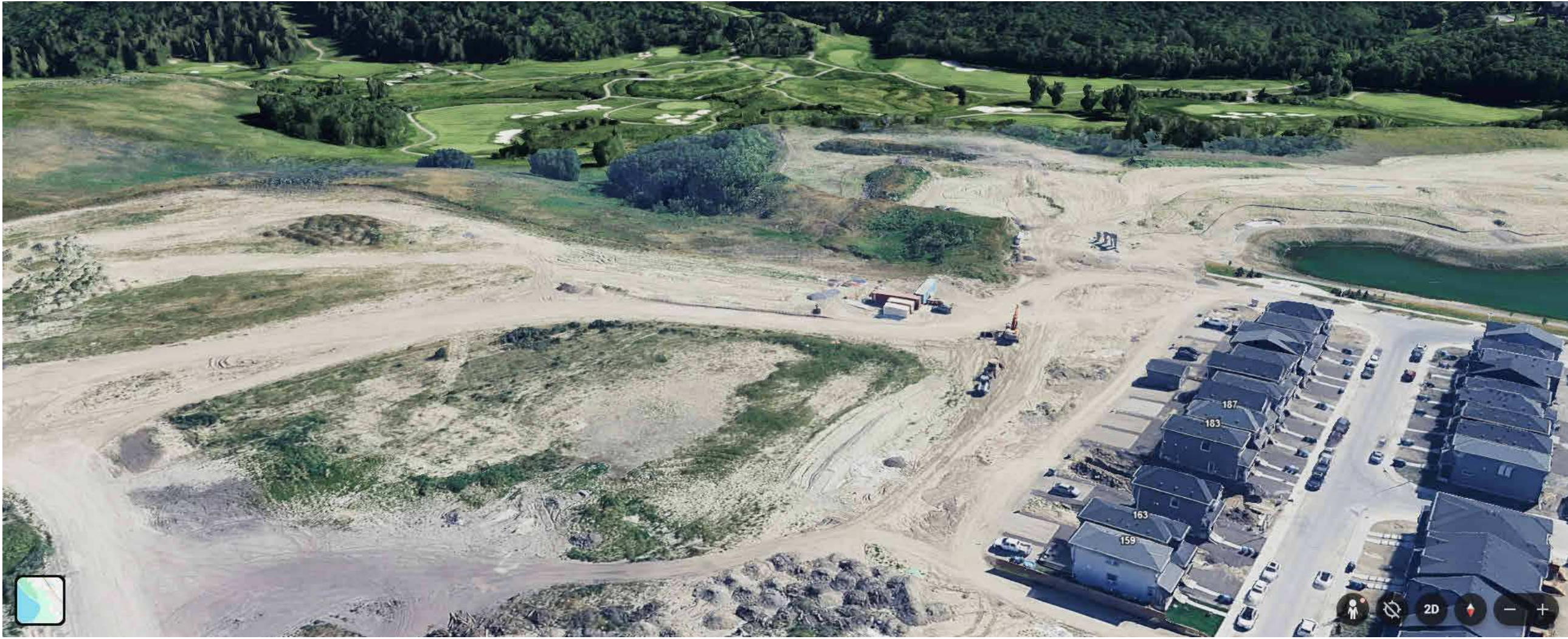
SITE PHOTO - SOUTH
