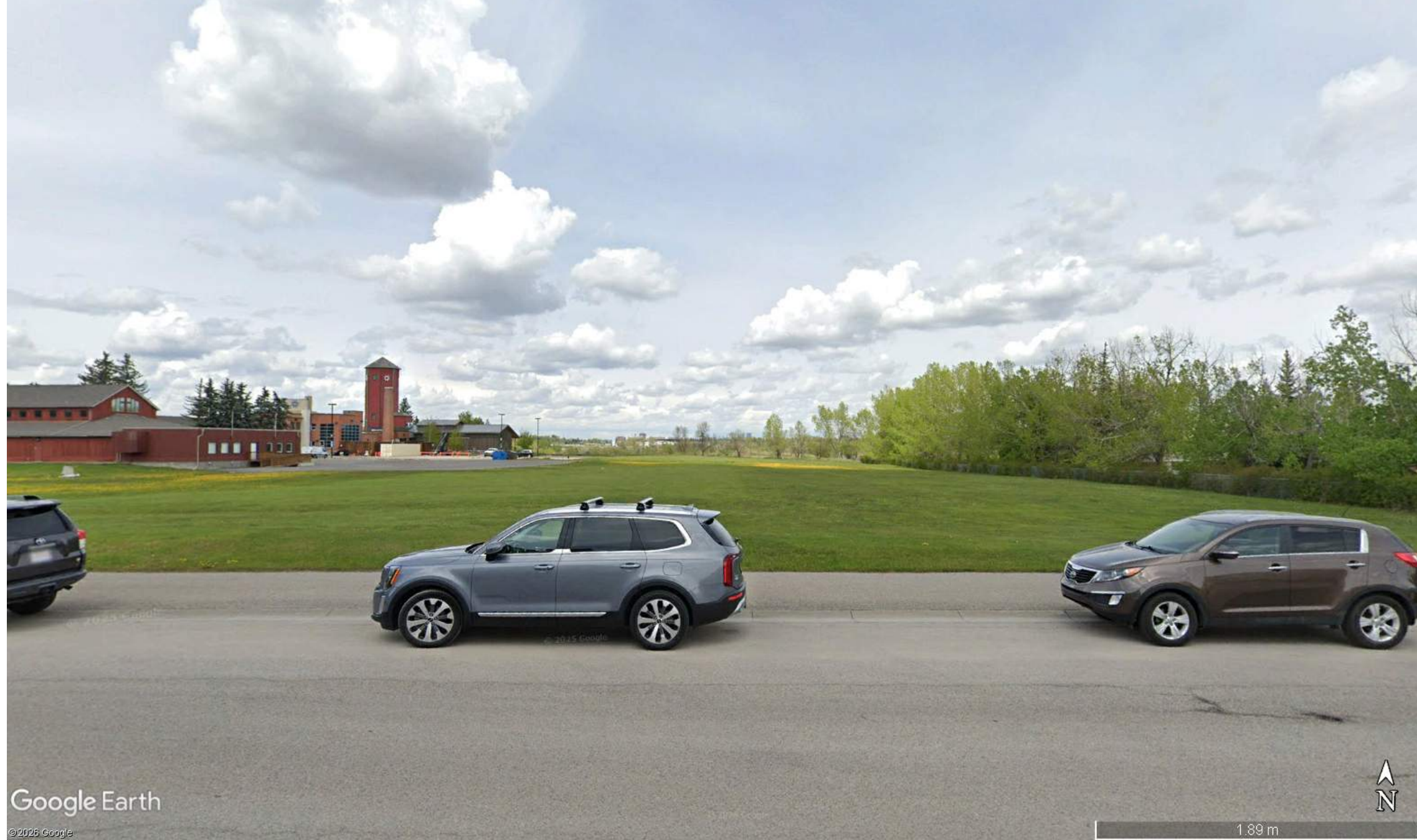
4- SOUTH VIEW (FROM 146 AVE SE)
