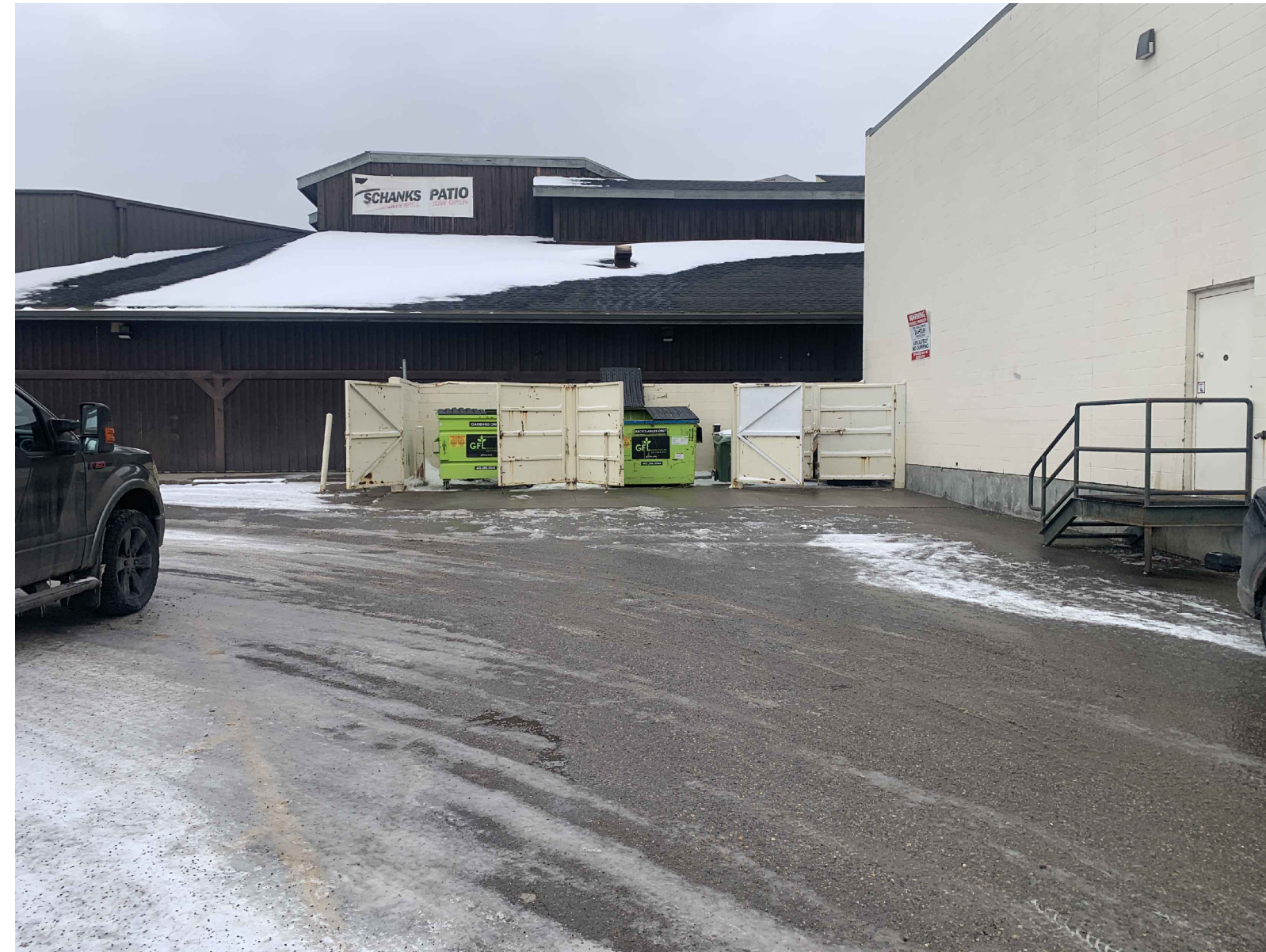
EXISTING ENCLOSURE VIEW FROM THE SOUTH
