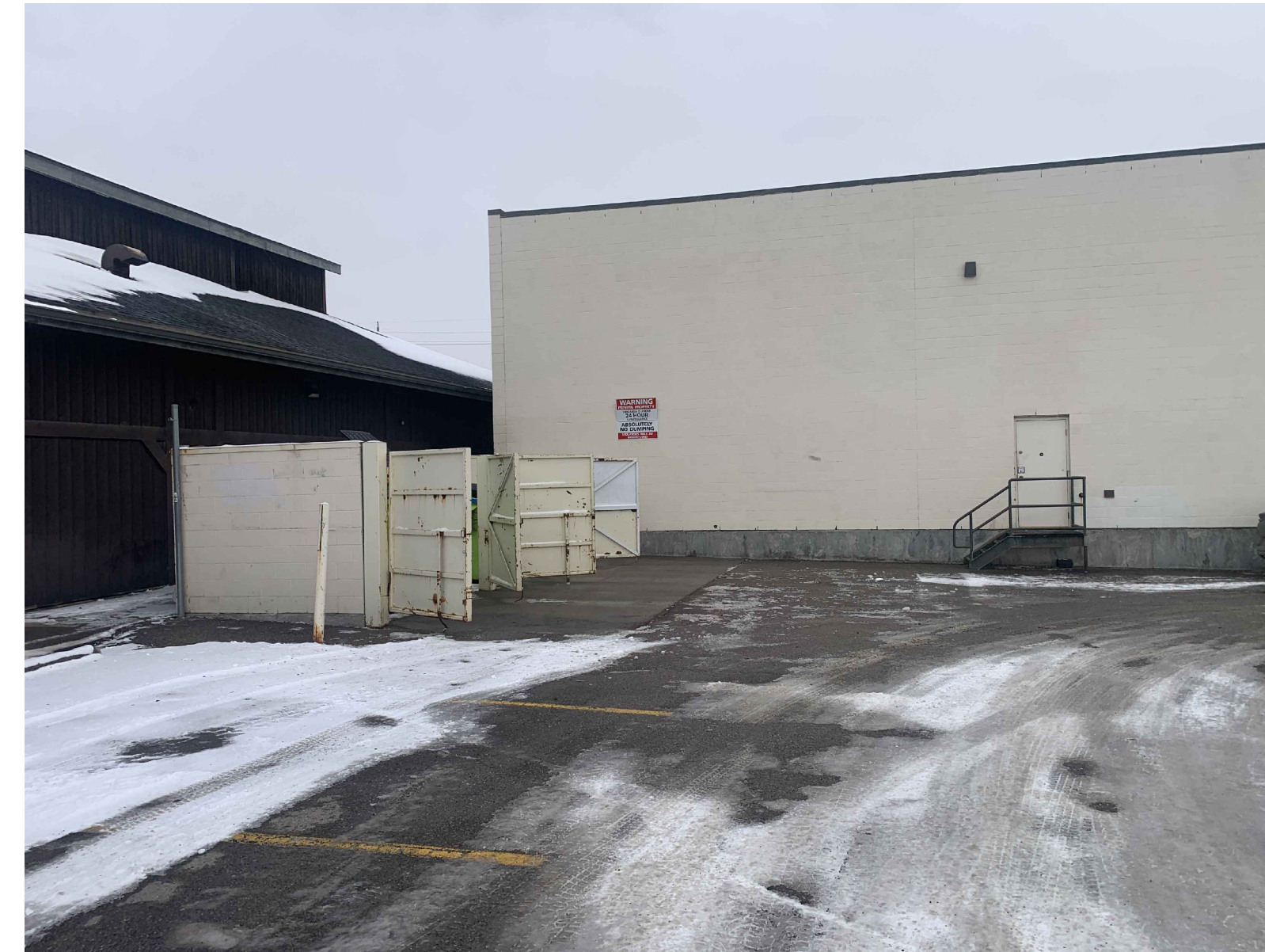
EXISTING ENCLOSURE VIEW FROM THE WEST
