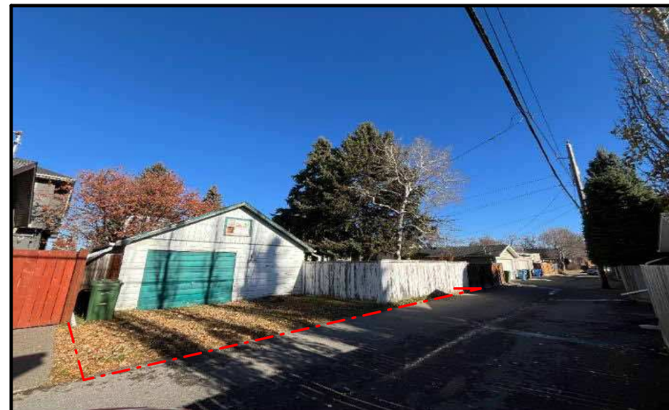
IMAGE 5: REAR PROPERTY FROM LANE + O/H POLE CONNECTION
