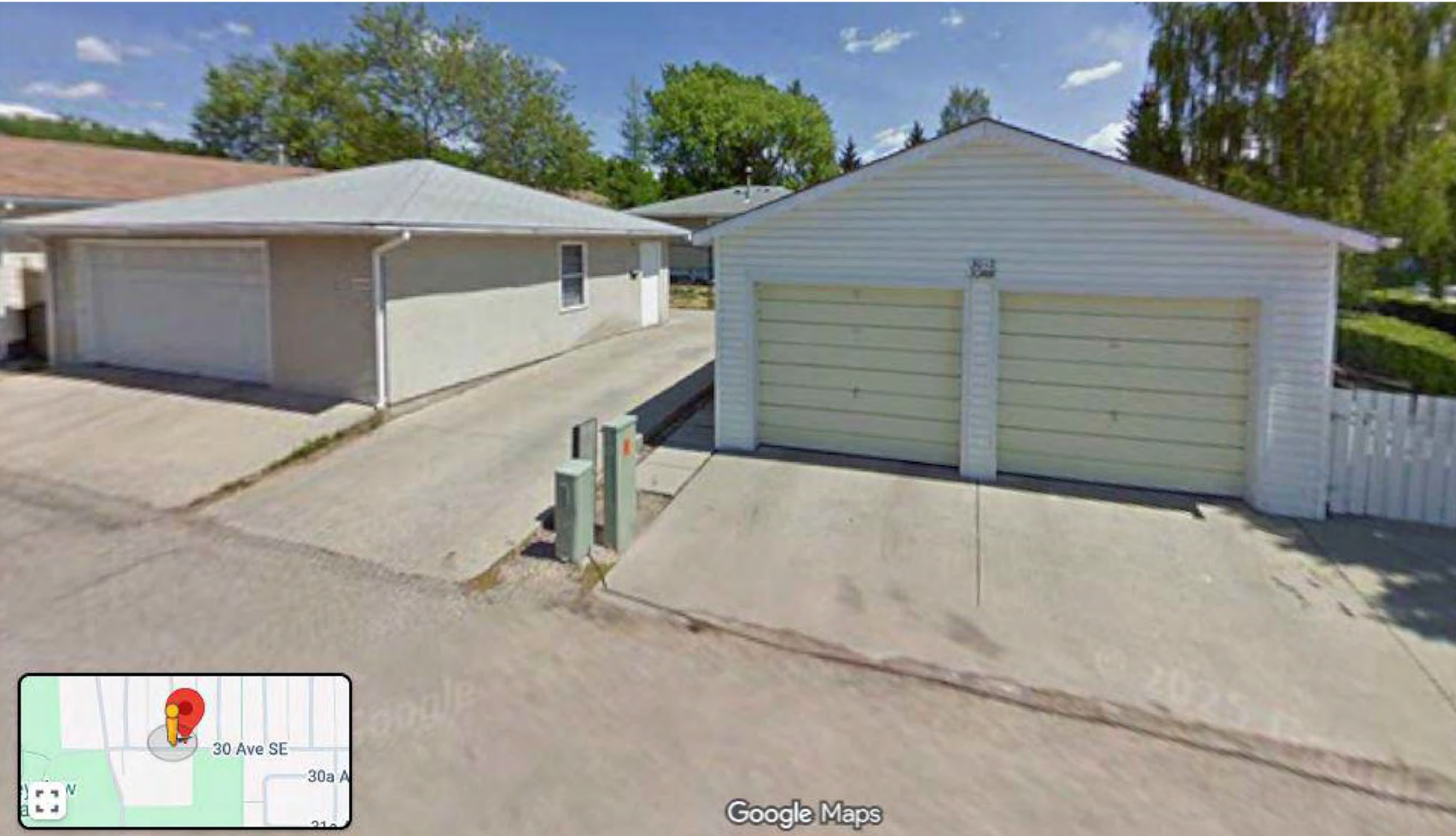
REAR OF SUBJECT PROPERTY AND NEIGHBOUR
