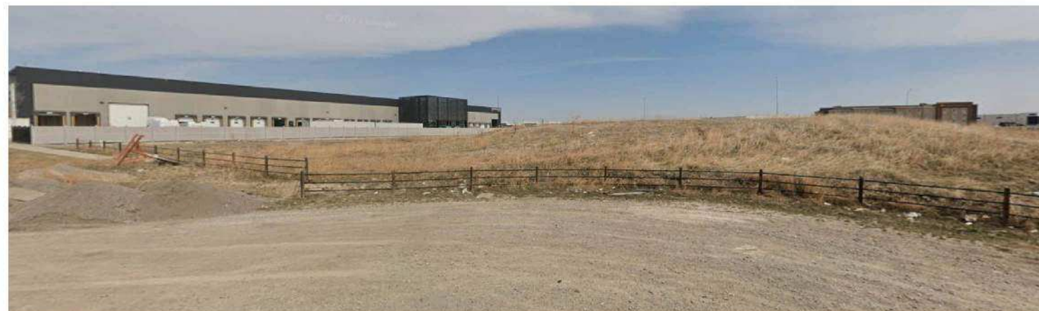
PIC. #2: PROJECT SOUTHWEST CORNER OF SITE AT END OF EXISTING ROAD. LOOKING NORTH TOWARDS EXISTING KINGSWOOD CABINETS BUILDING.
