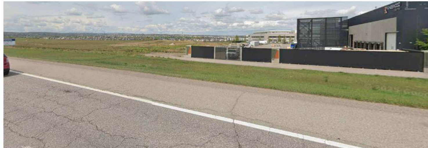
PIC. #3: PROJECT NORTHEAST CORNER OF SITE FROM DEERFOOT TRAIL. EXISTING KINGSWOOD CABINETS BUILDING YARD ON THE RIGHT.
