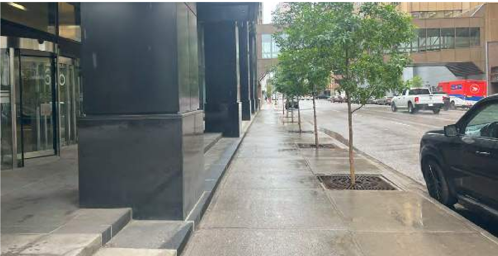
4 - SW CORNER - COLUMNS IN FRONT OF THE MAIN ENTRANCE TO THE BUILDING
