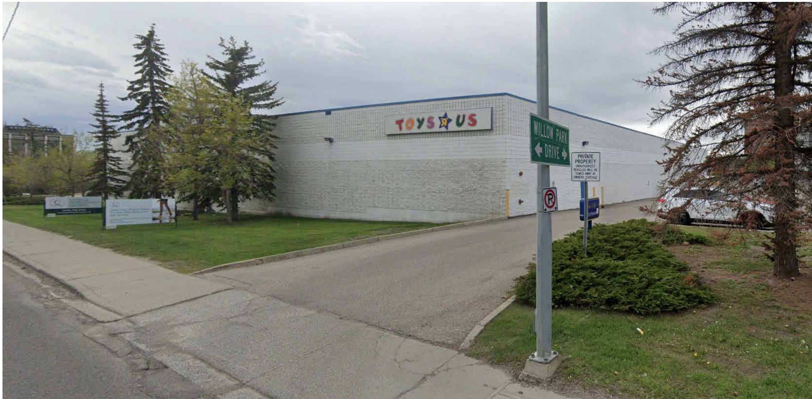
EXISTING BUILDING CONDITION NORTH-EAST ALONG BONAVENTURE DR SE
