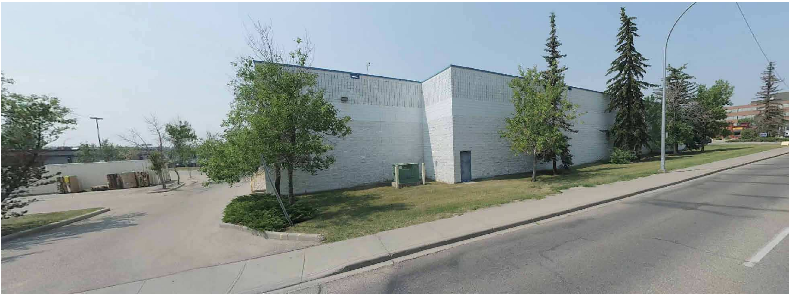
EXISTING BUILDING CONDITION SOUT-EAST ALONG BONAVENTURE DR SE
