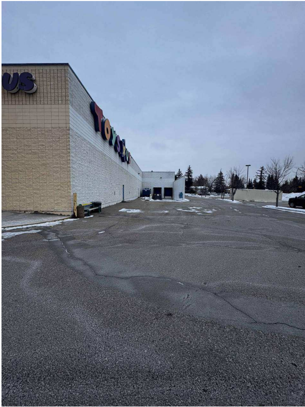
EXISTING BUILDING CONDITION SOUTH-WEST CORNER
