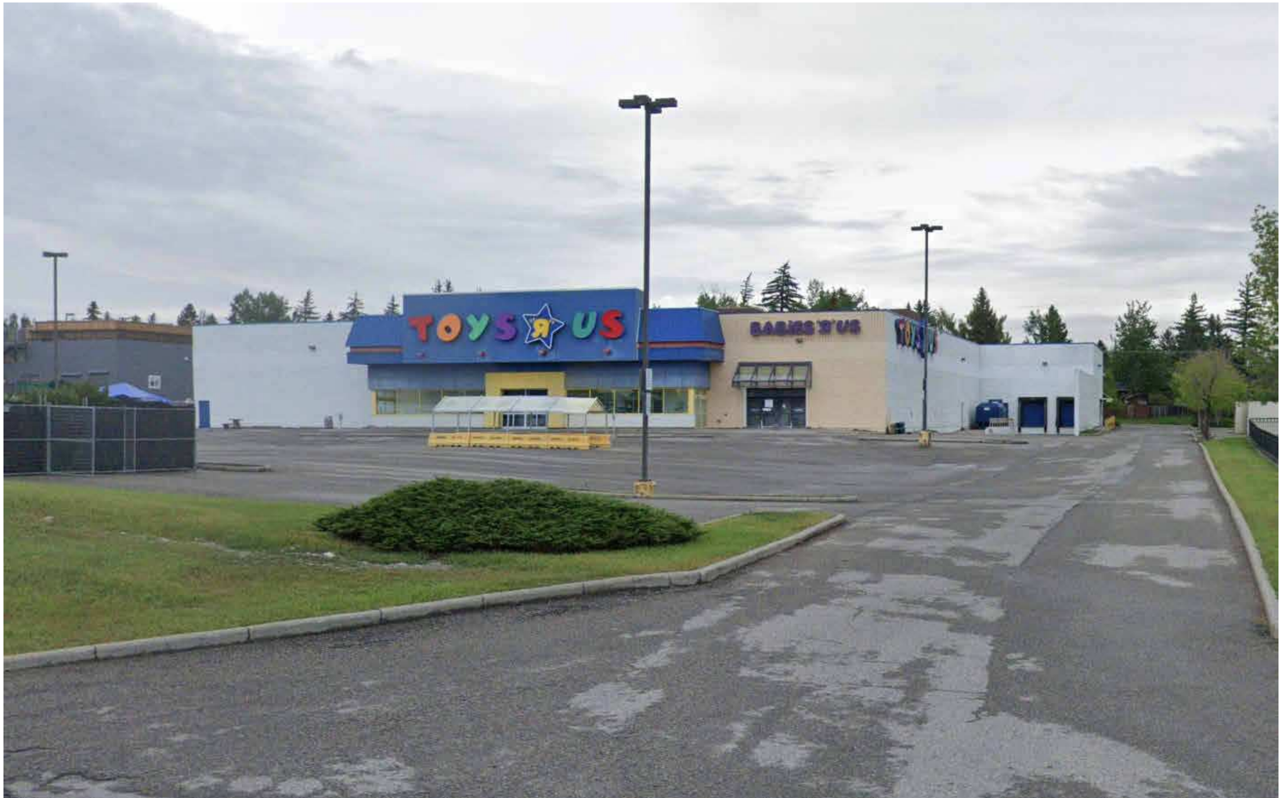
EXISTING BUILDING CONDITION SOUTH-WEST ALONG MACLEOD TRAIL
