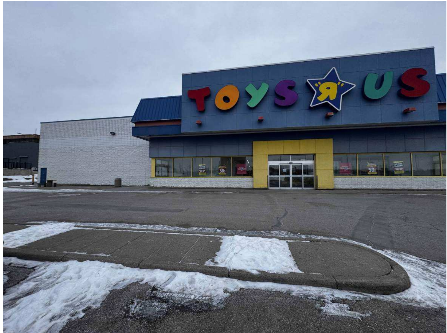
EXISTING BUILDING CONDITION WEST (NORTH WING)
