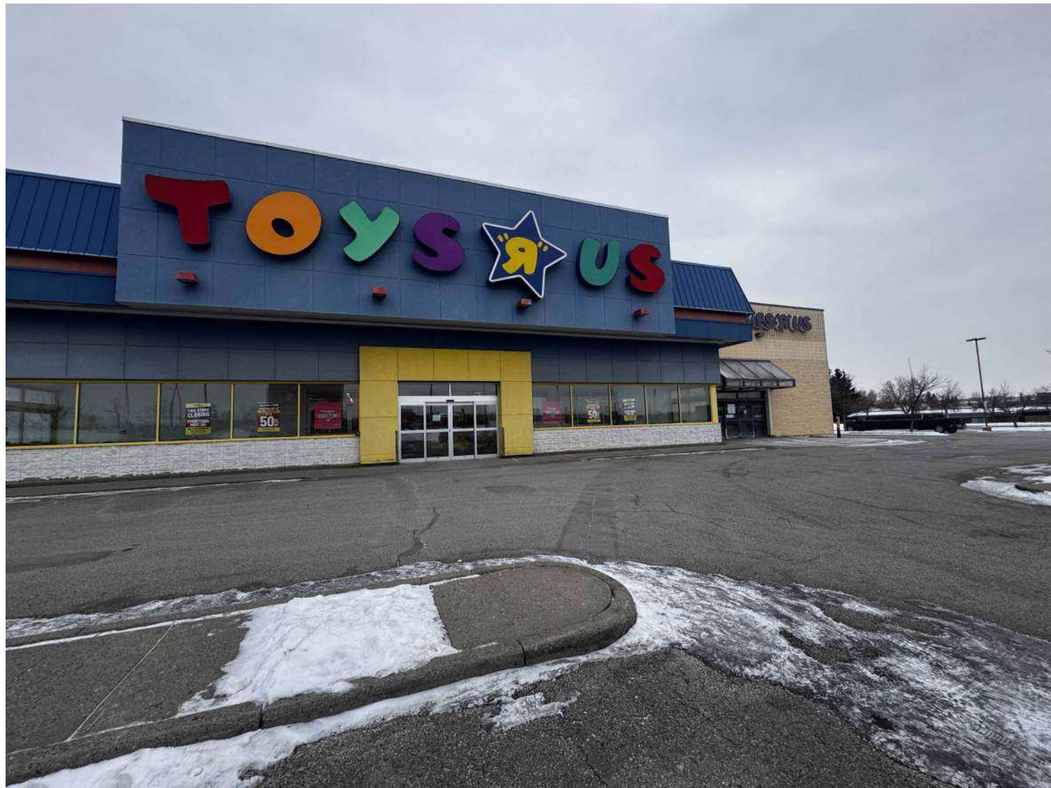
EXISTING BUILDING CONDITION WEST (SOUTH WING)
