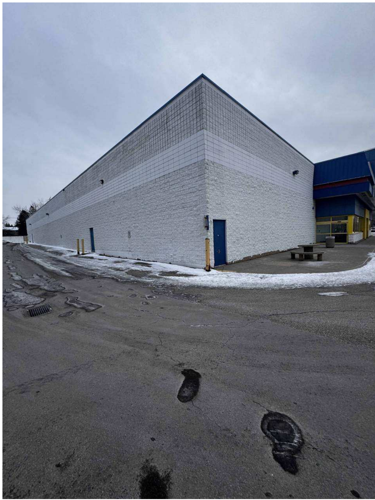
EXISTING BUILDING CONDITION NORTH-WEST CORNER
