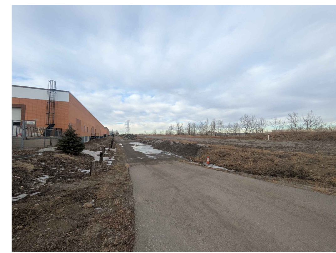
3 DP01 PHOTO - VIEW FROM THE SW N/A
