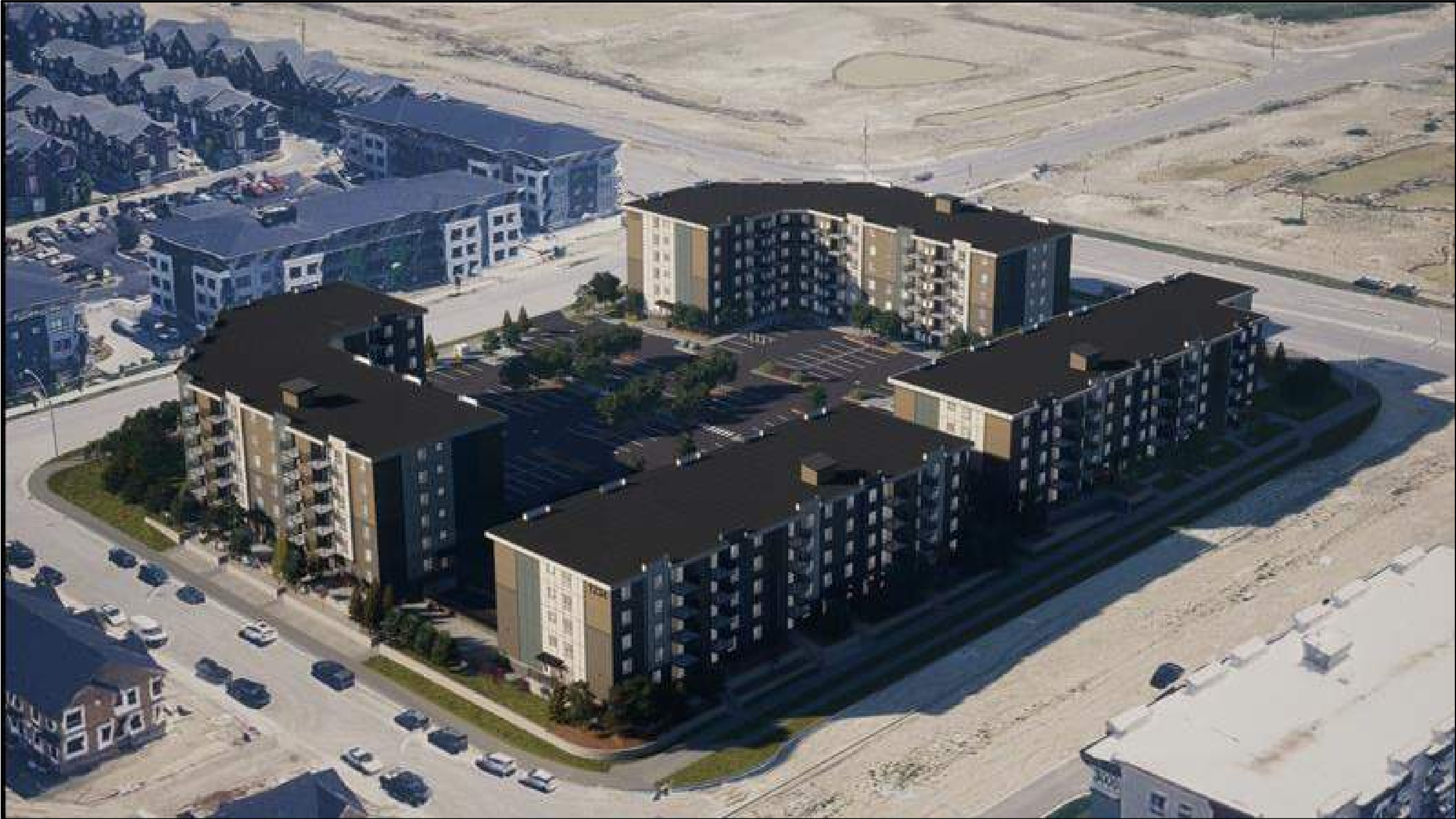
NORTH WEST CORNER
