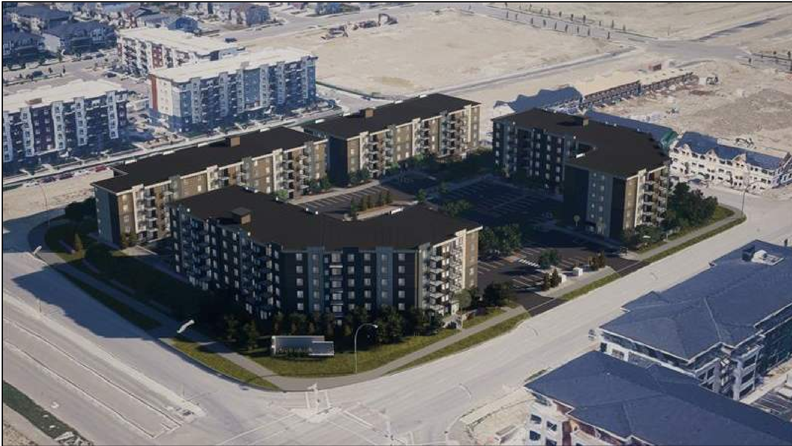
SOUTH EAST CORNER
