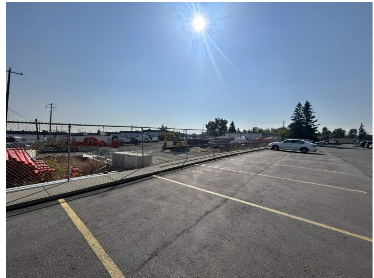
IMAGE 11: View of west corner from the parking lot west of the site.
