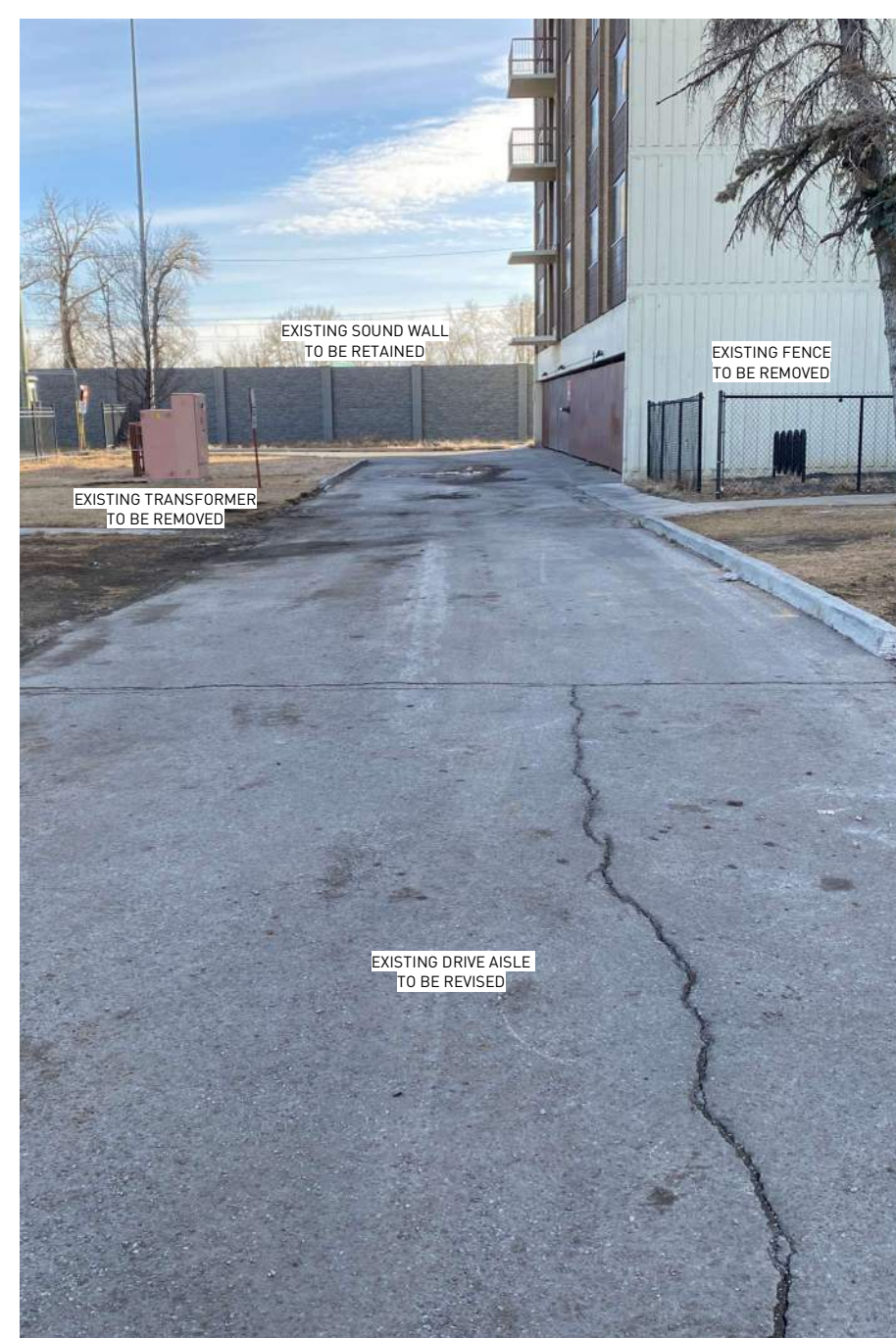
EXISTING SITE PHOTO 10: FACING SOUTH
