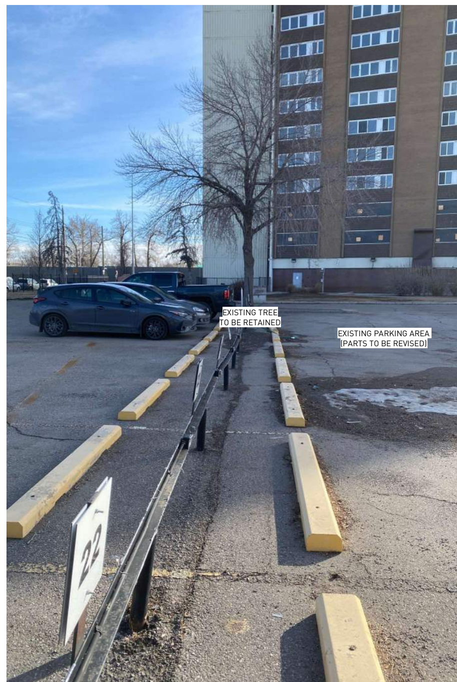
EXISTING SITE PHOTO 6: FACING SOUTH
