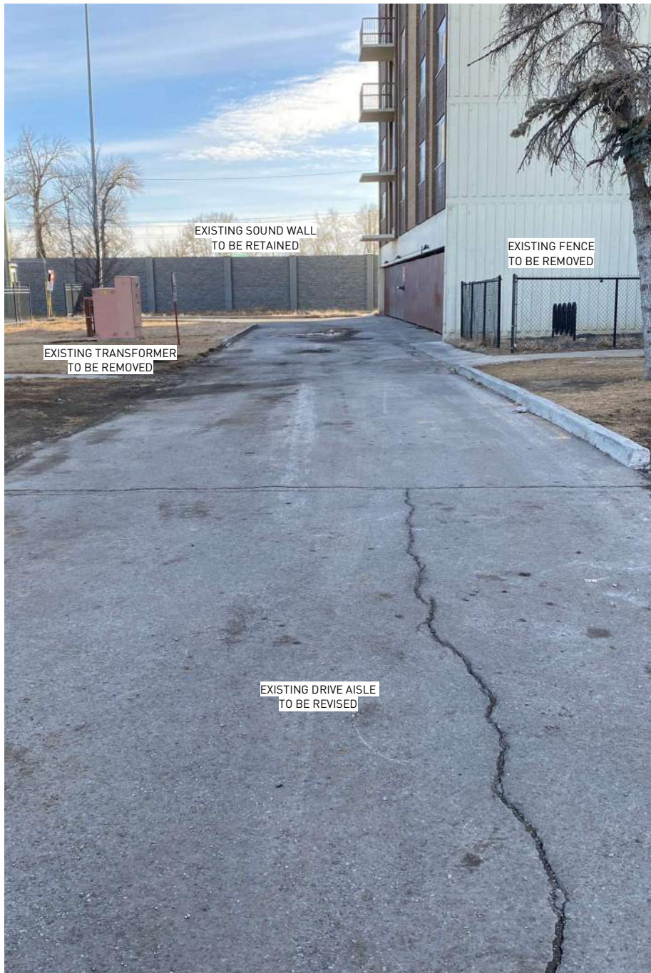
EXISTING SITE PHOTO 10: FACING SOUTH
