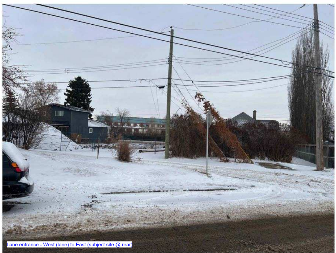
Lane entrance - West (lane) to East (subject site @ rear)
