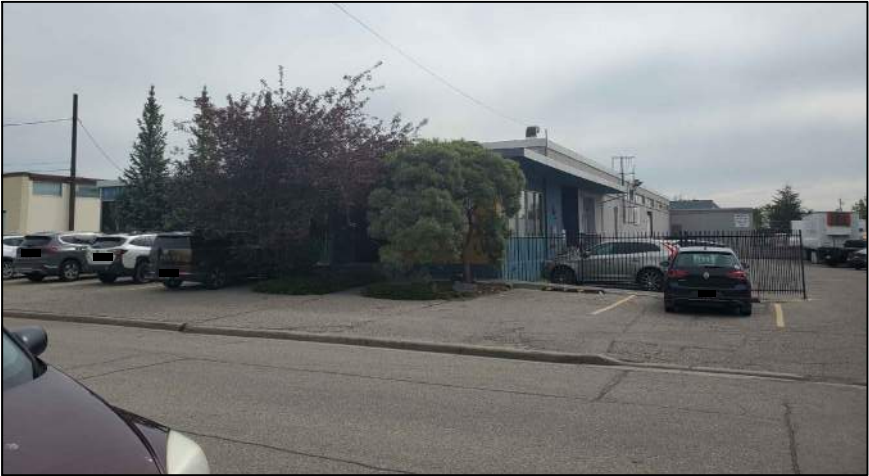
FRONT (WEST) ELEVATION - ENTRANCE
