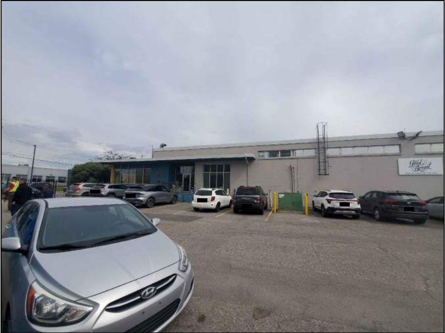
SOUTH ELEVATION - WEST PORTION
