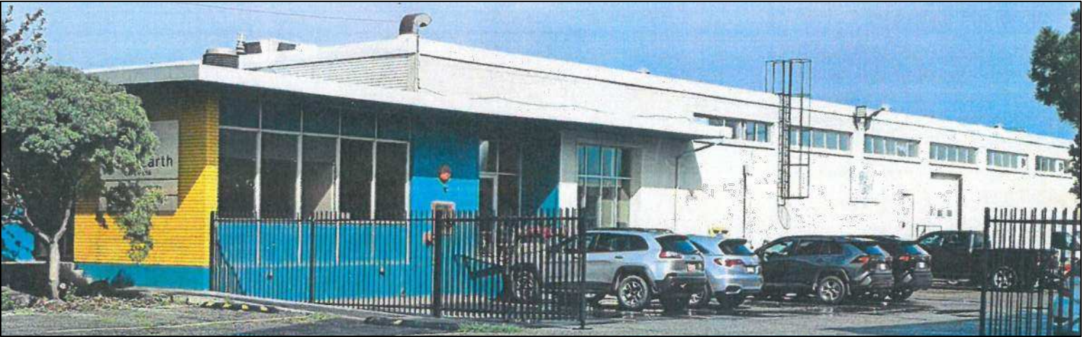
FRONT (WEST) AND SOUTH ELEVATIONS
