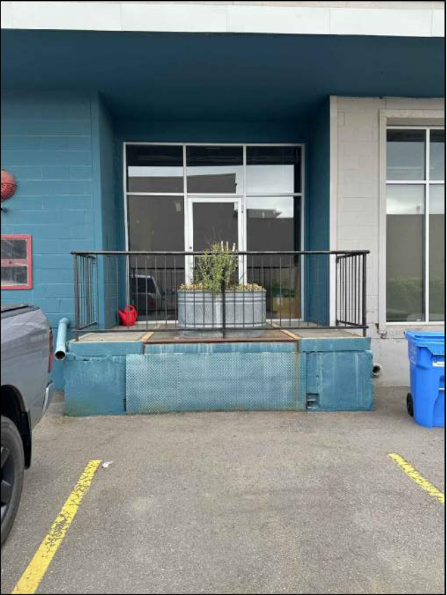
EXTERIOR OF EXISTING CURTAIN WALL AND FORMER LOADING DOCK TO BE REMOVED TO ACCOMMODATE NEW LOADING DOOR AND ELEVATING DOCK LIFT
