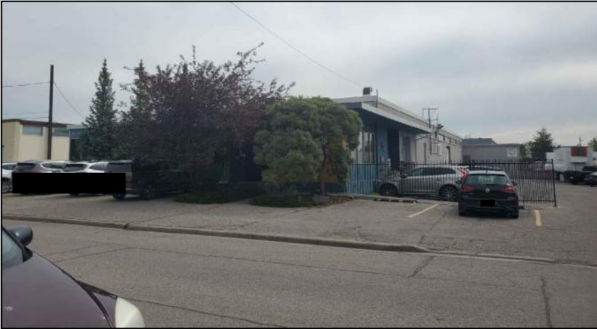
FRONT (WEST) ELEVATION - ENTRANCE
