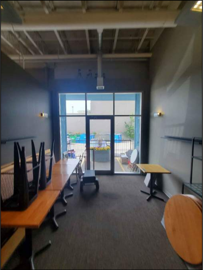
INTERIOR OF EXISTING CURTAIN WALL TO BE REMOVED TO ACCOMMODATE NEW LOADING DOOR ON SOUTH WALL
