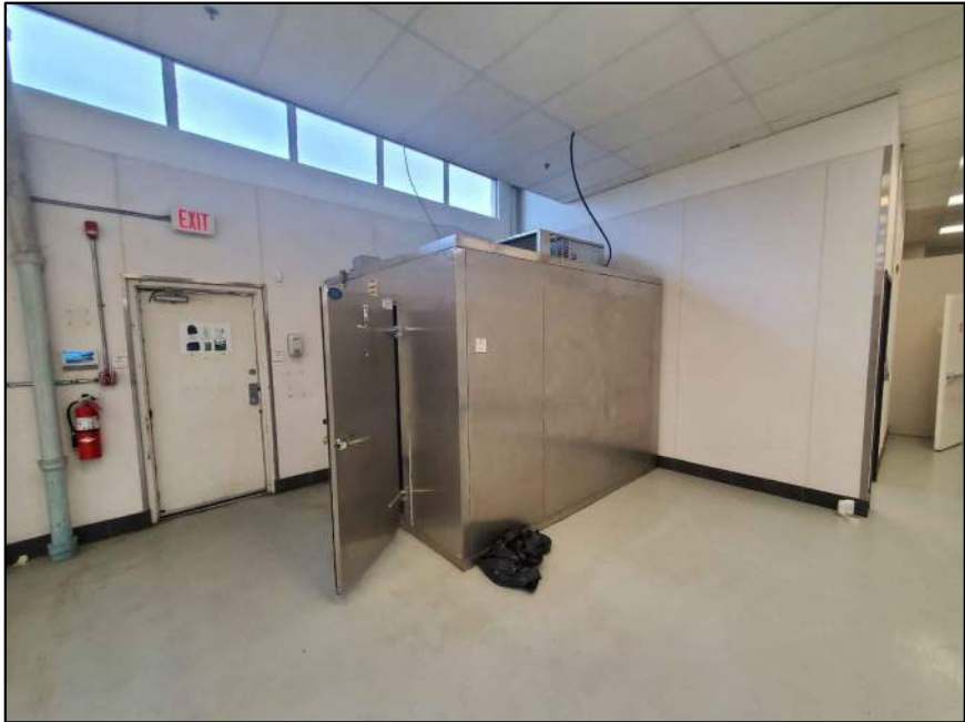
INTERIOR OF SOUTH ELEVATION - EXISTING FREEZER TO BE RELOCATED
