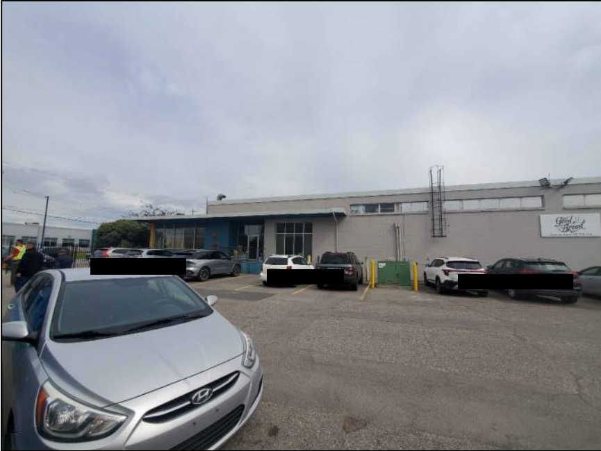
SOUTH ELEVATION - WEST PORTION
