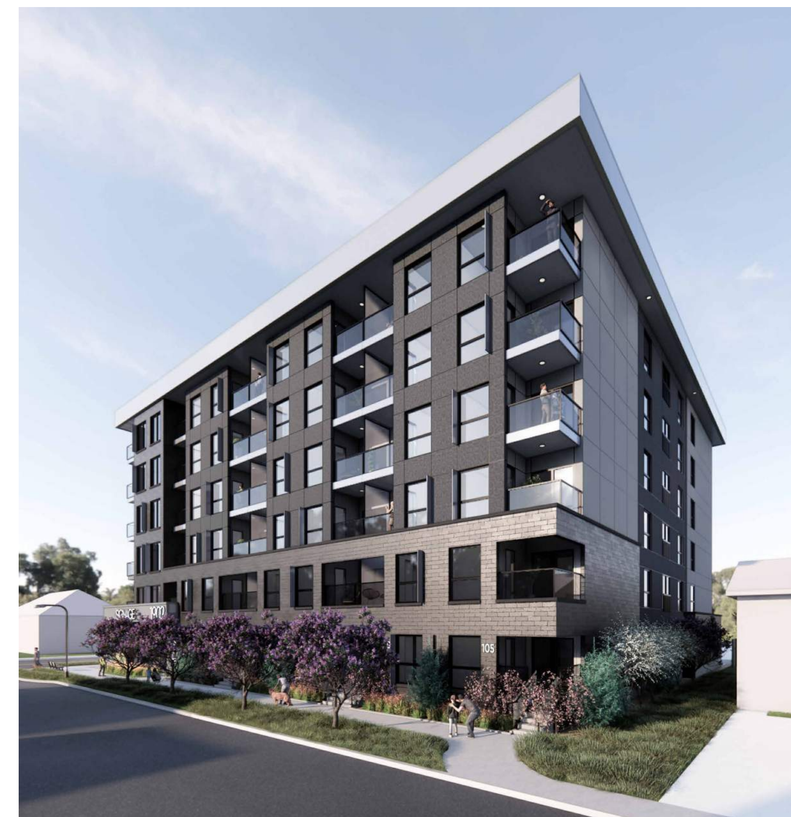
SW VIEW - 24A STREET SW FRONTAGE
