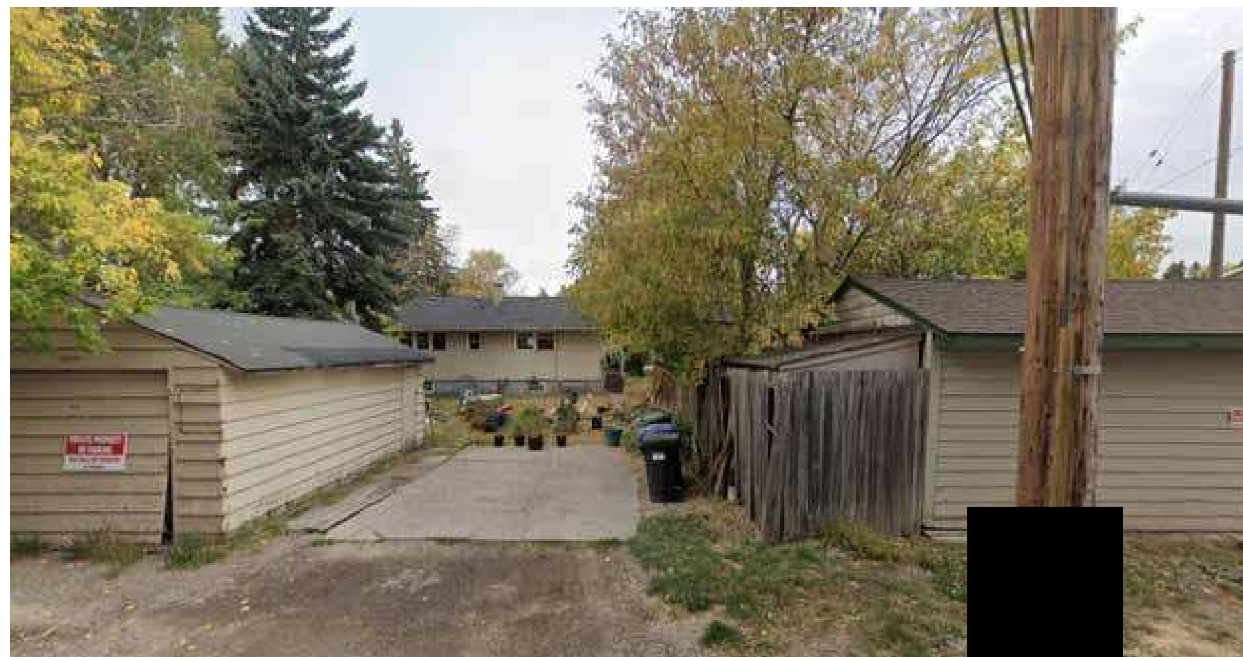
S7 - SITE PHOTO - VIEW FROM EAST
