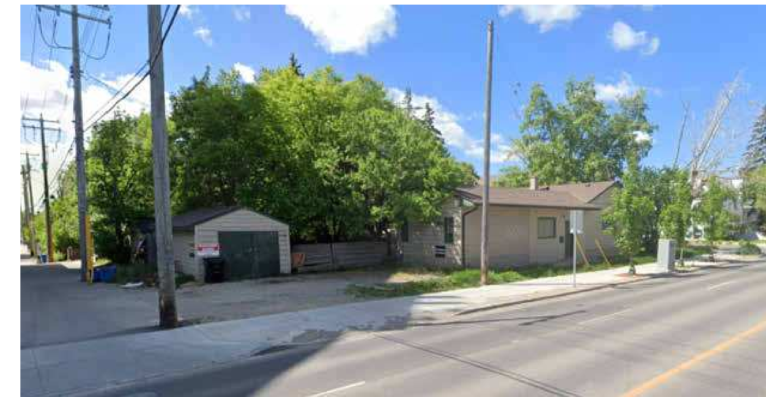
S6 - SITE PHOTO - VIEW FROM NORTHEAST
