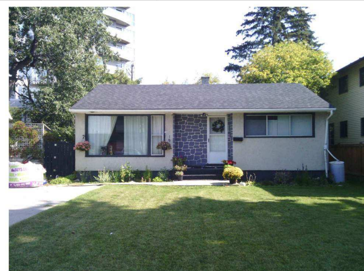
PHOTO 2 (1906 24A STREET SW)
