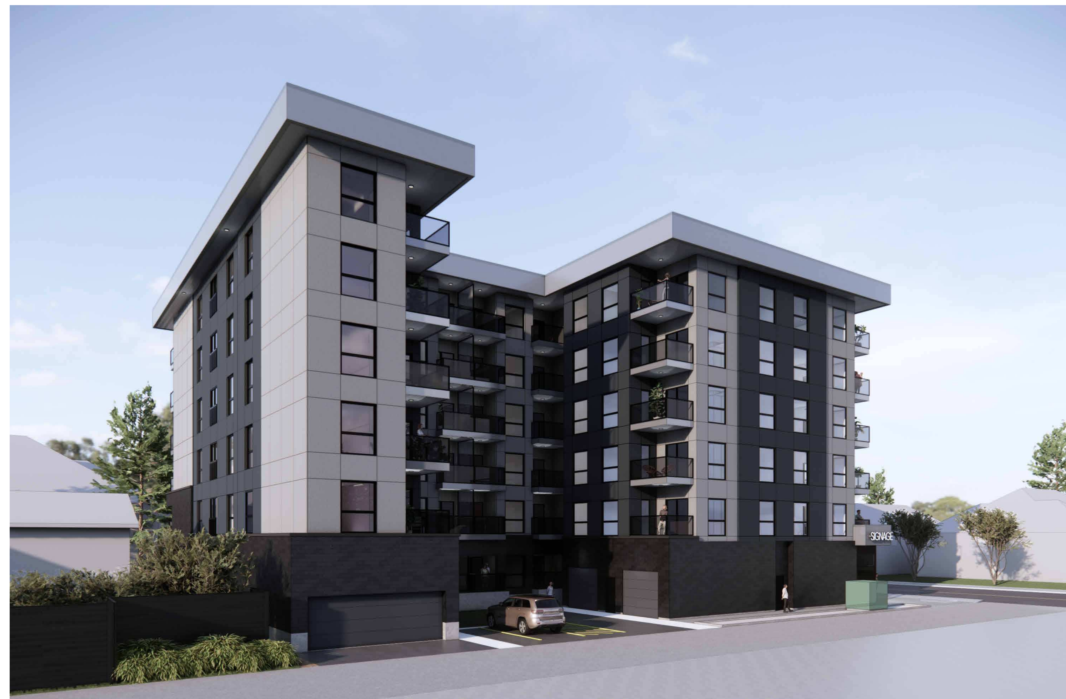
SE VIEW - FROM LANE
