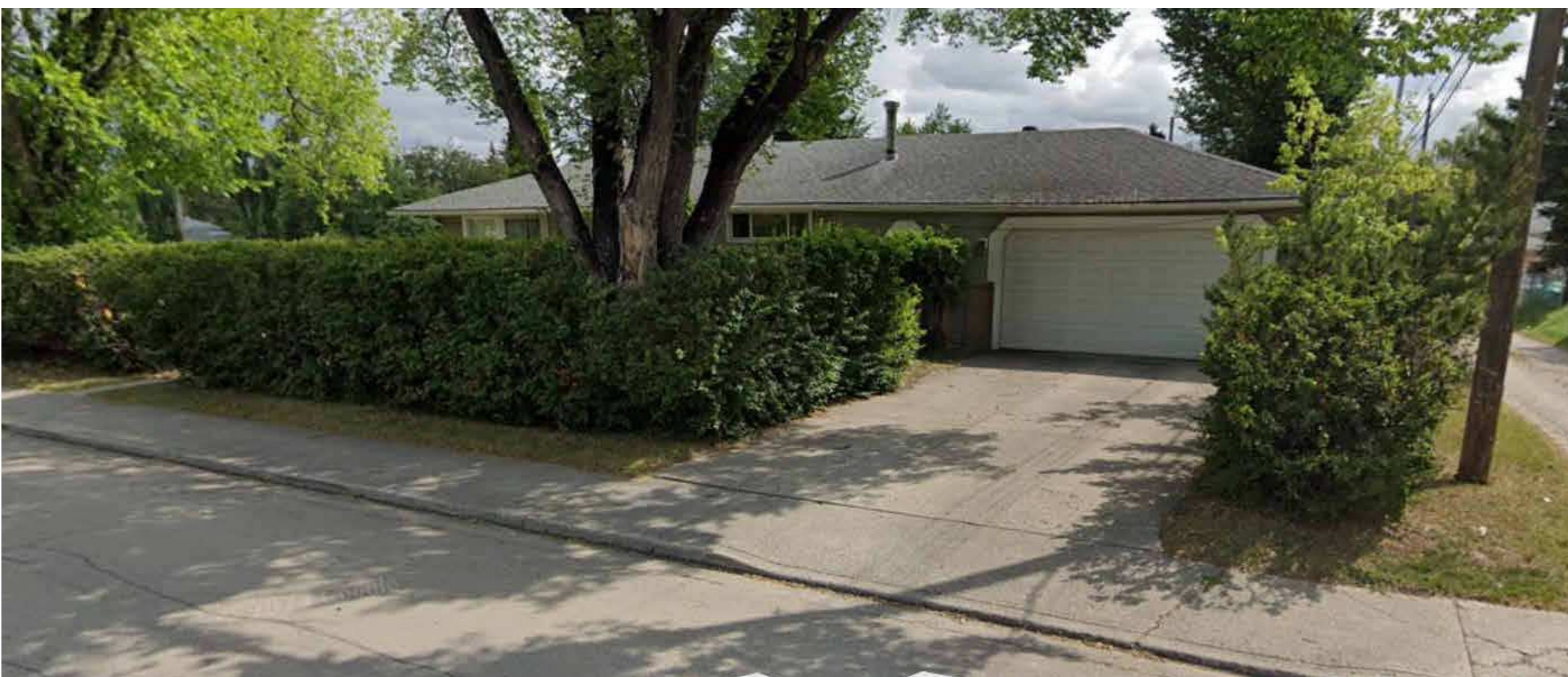
1 VIEW FROM 43 STREET S.W.
