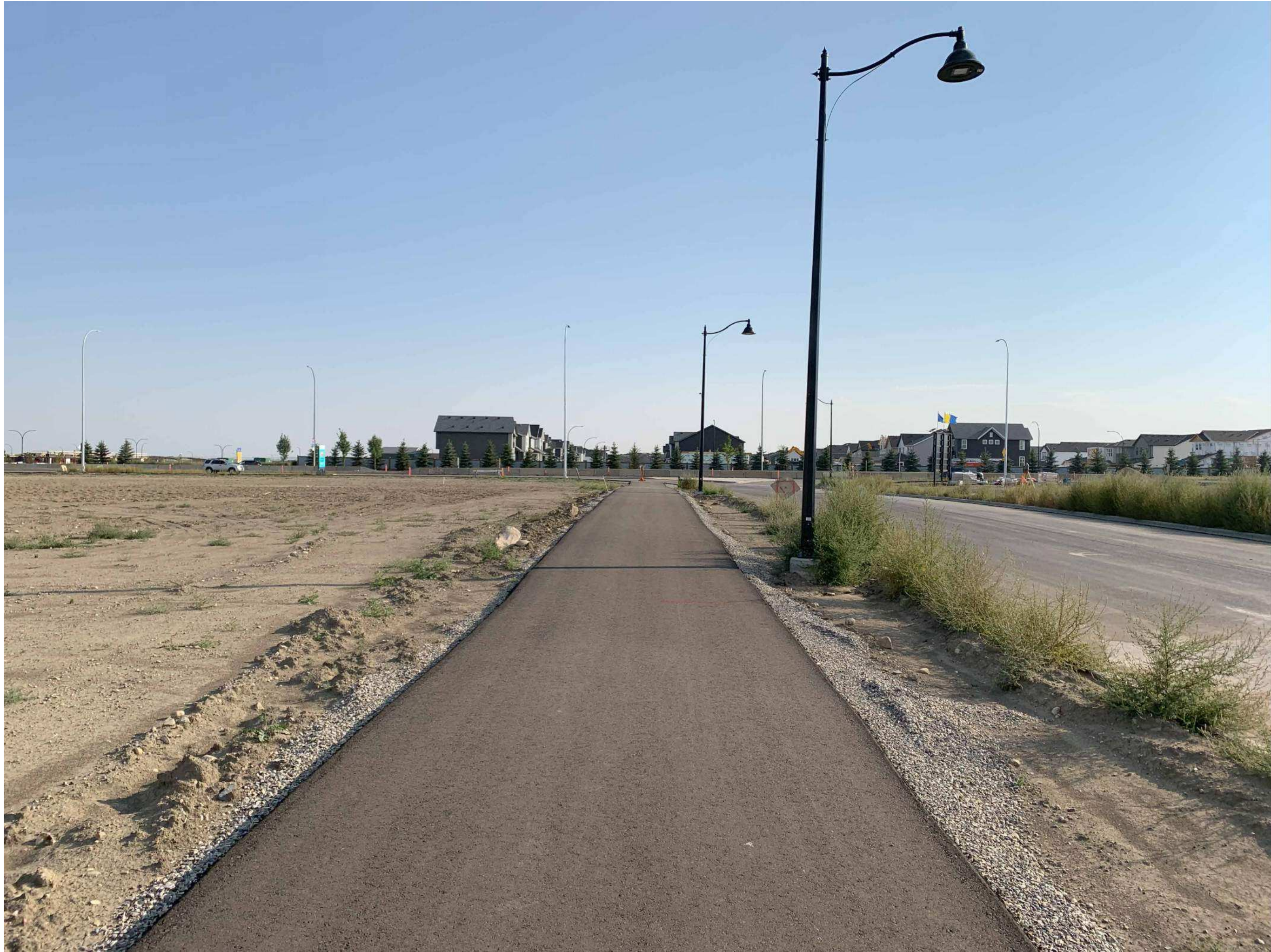
1 SITE PHOTO (S to W) A6.0
