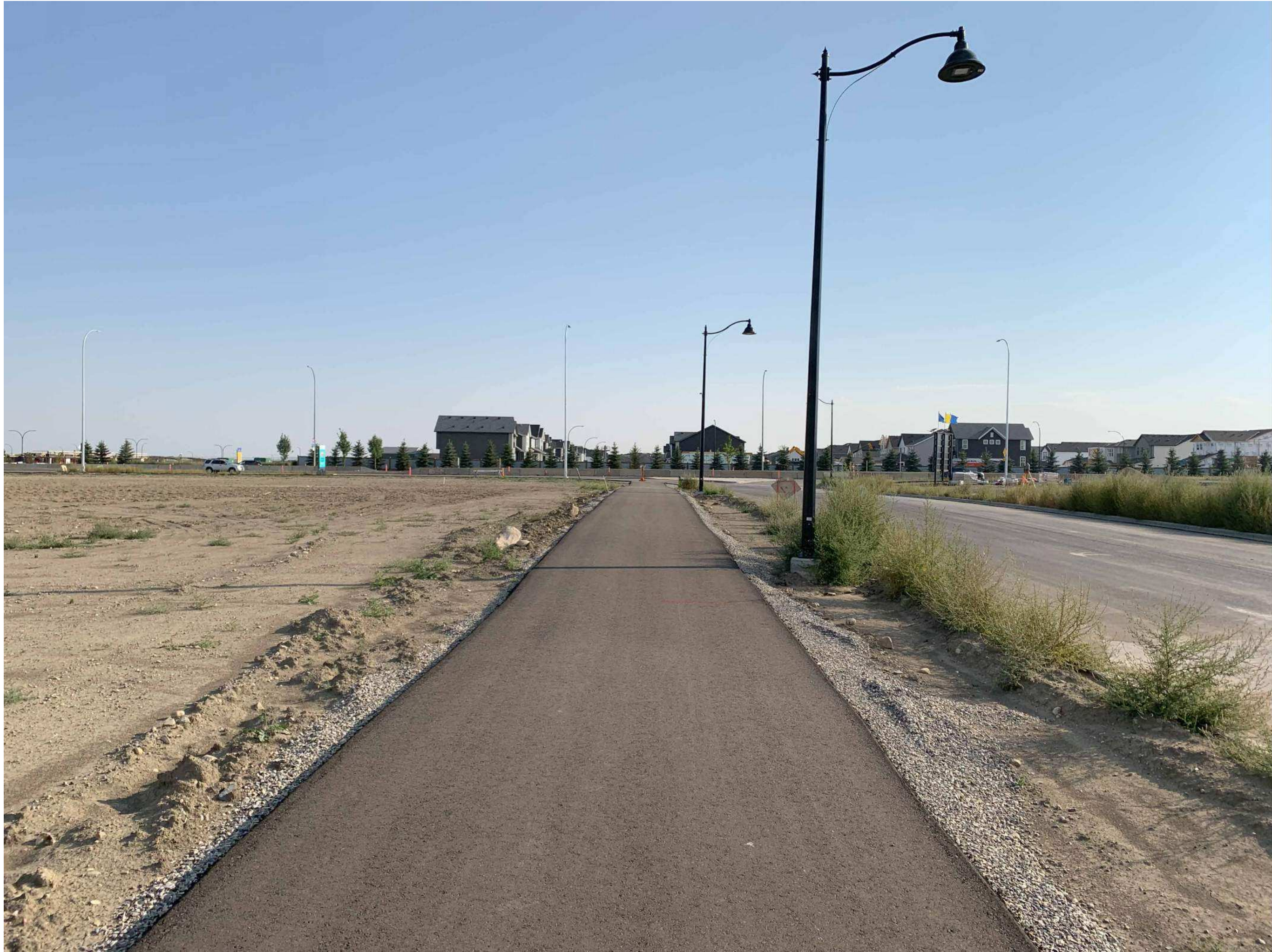
1 SITE PHOTO (S to W) A6.0
