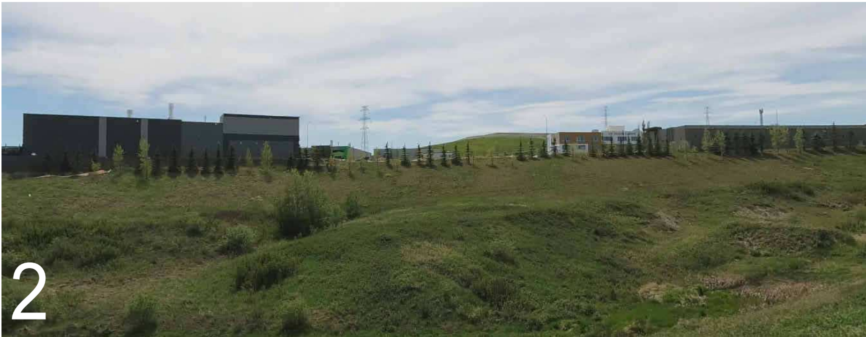
LOOKING SOUTHWEST TO SITE
