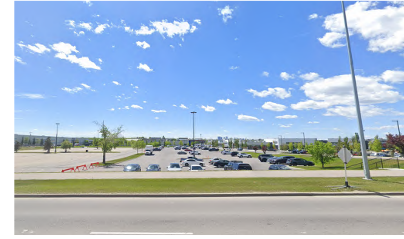
2 DP1.0 EXTERIOR SITE PHOTO SCALE: 1:8
