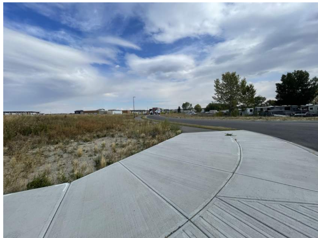
8 Street View - East DP0.03 SCALE:1:1000
