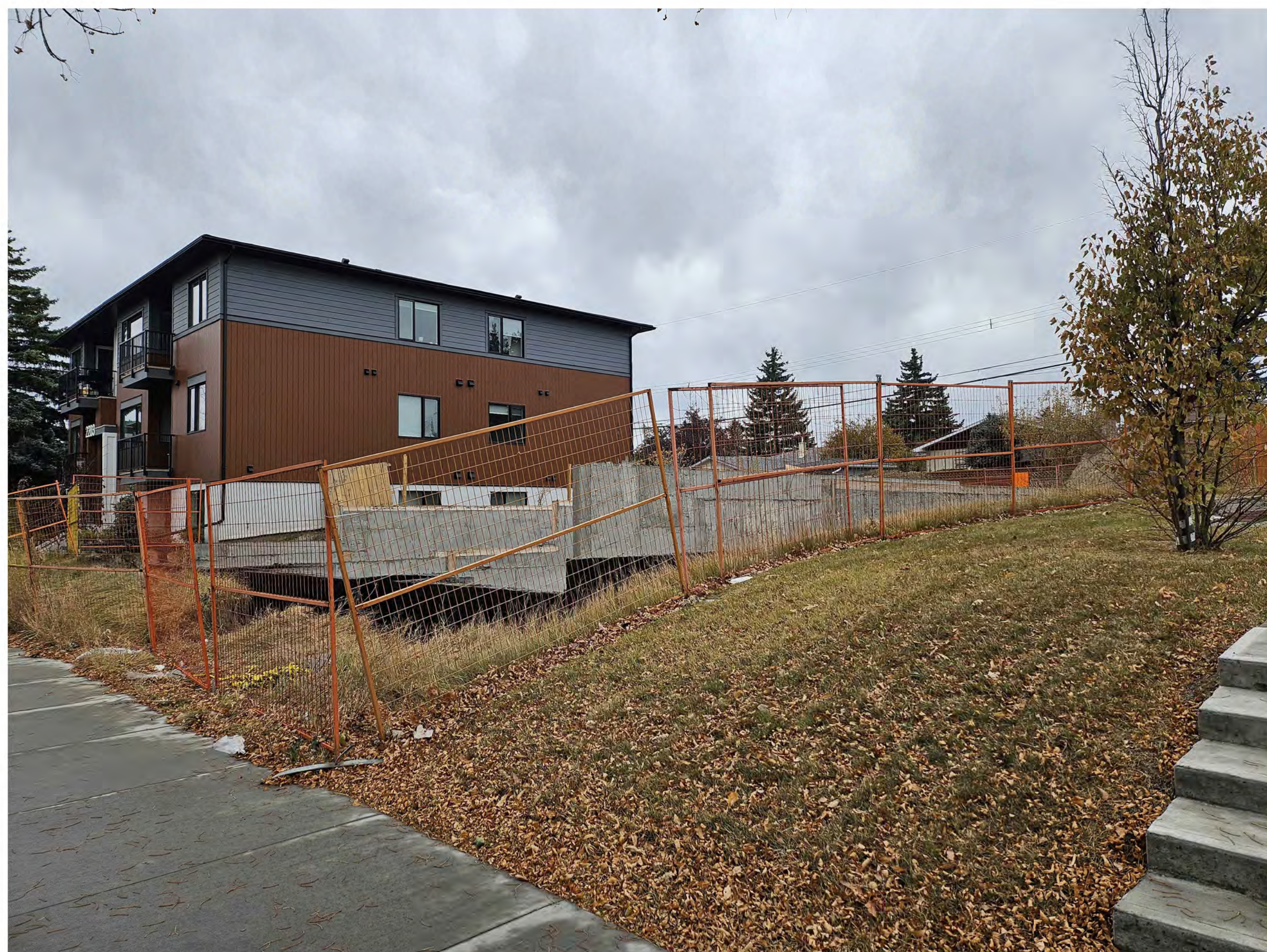
PROJECT SOUTH ADJACENT
