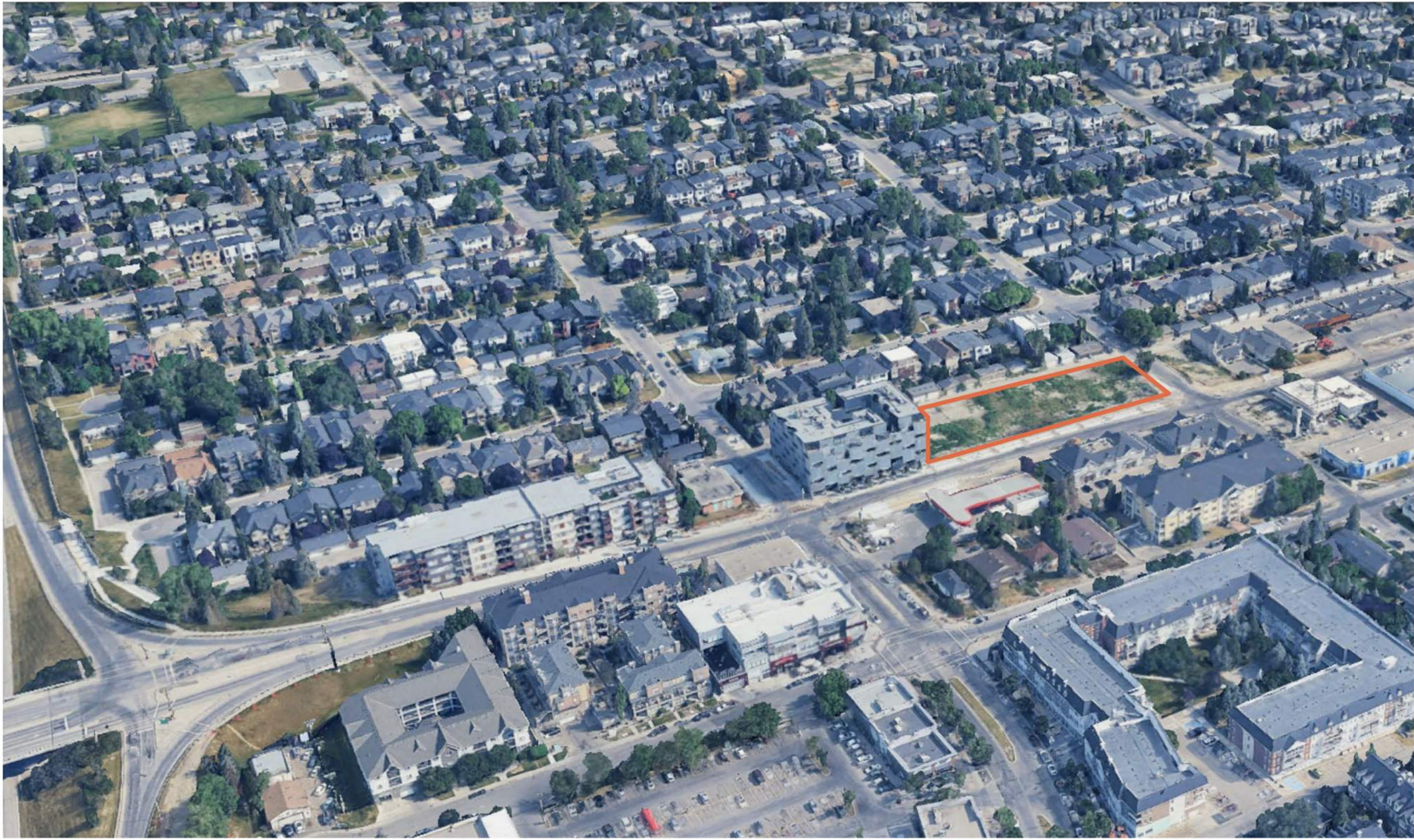
Aerial View from Southwest
