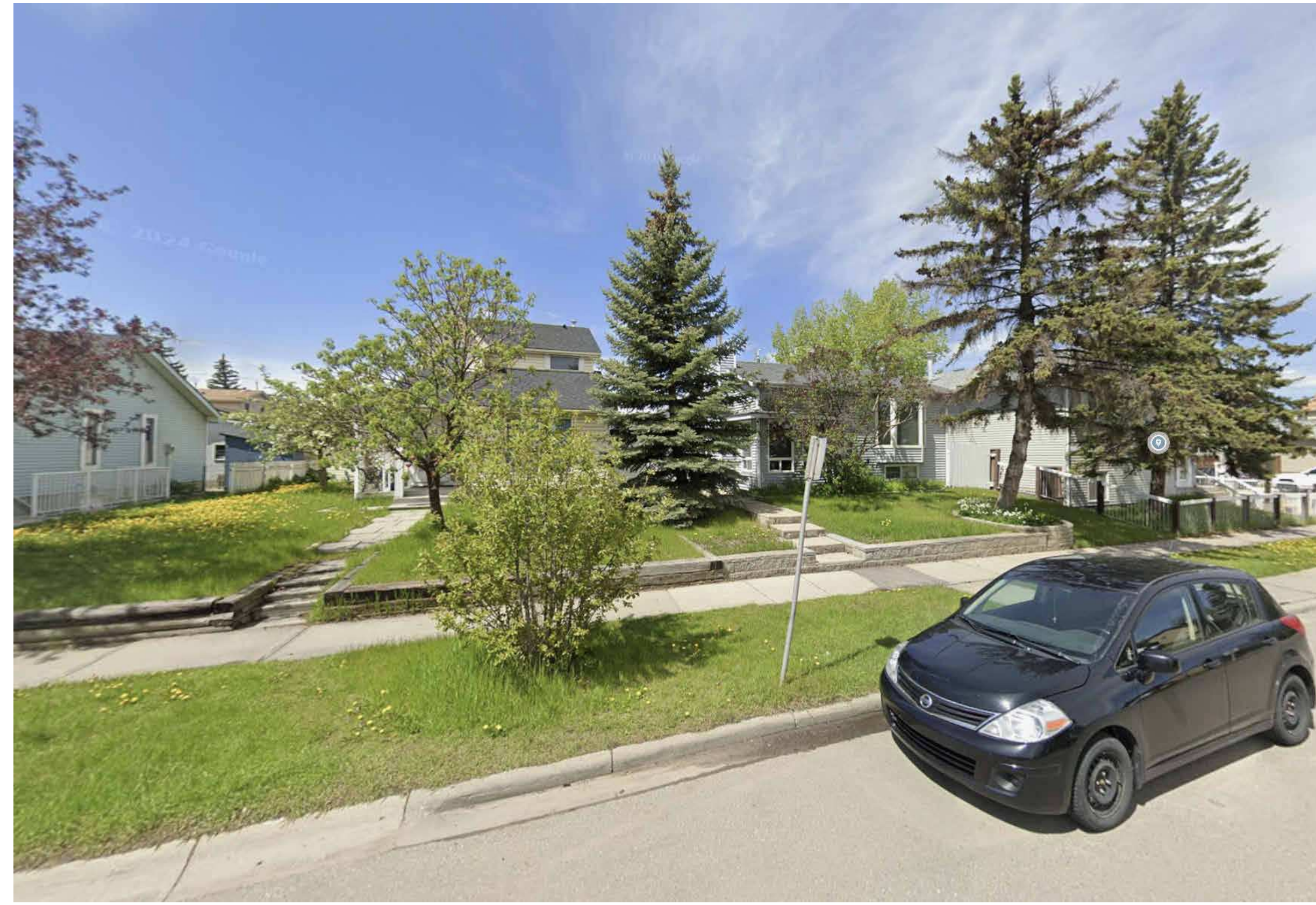
S1 | SITE PHOTO - VIEW FROM SOUTHEAST
