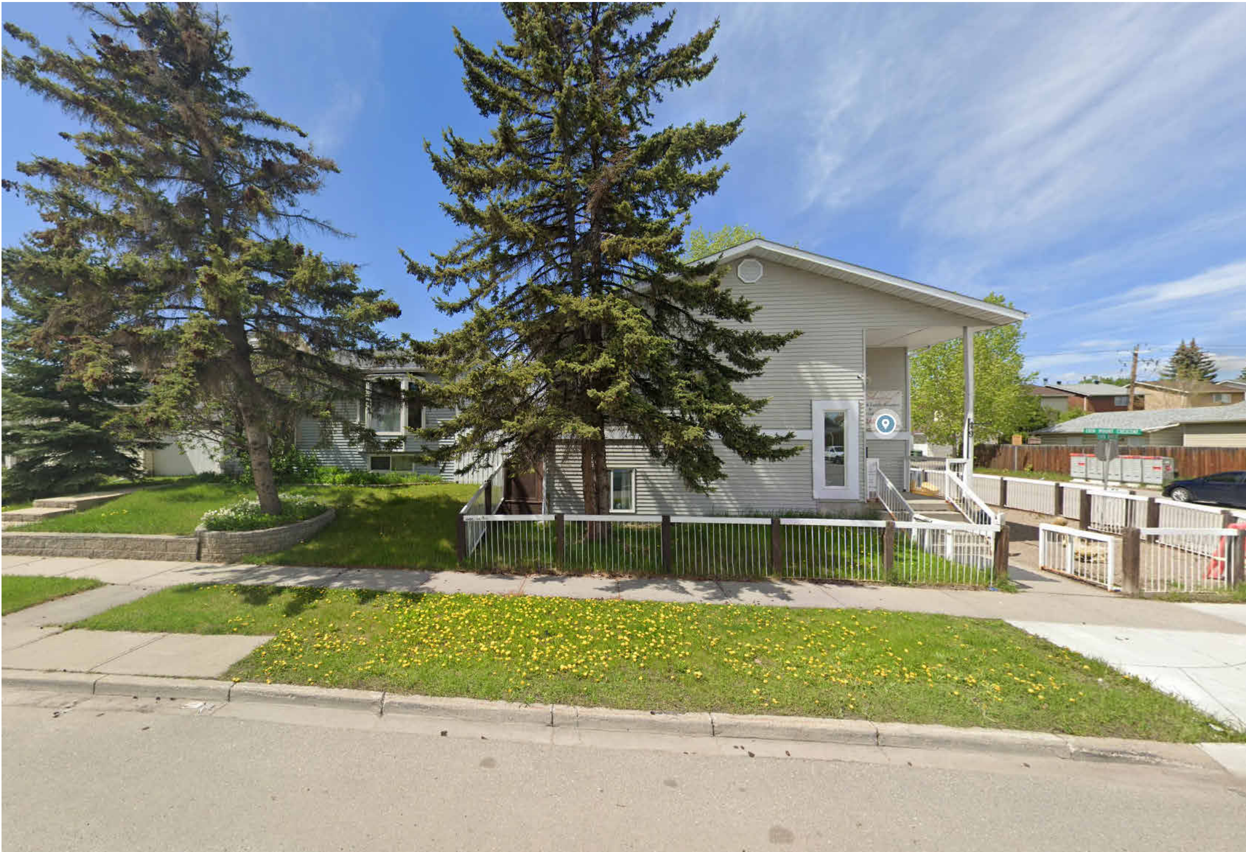
S2 | SITE PHOTO - VIEW FROM EAST
