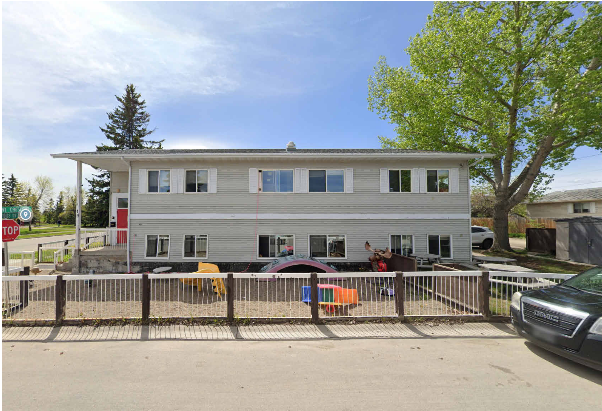
S6 | SITE PHOTO - VIEW FROM NORTH
