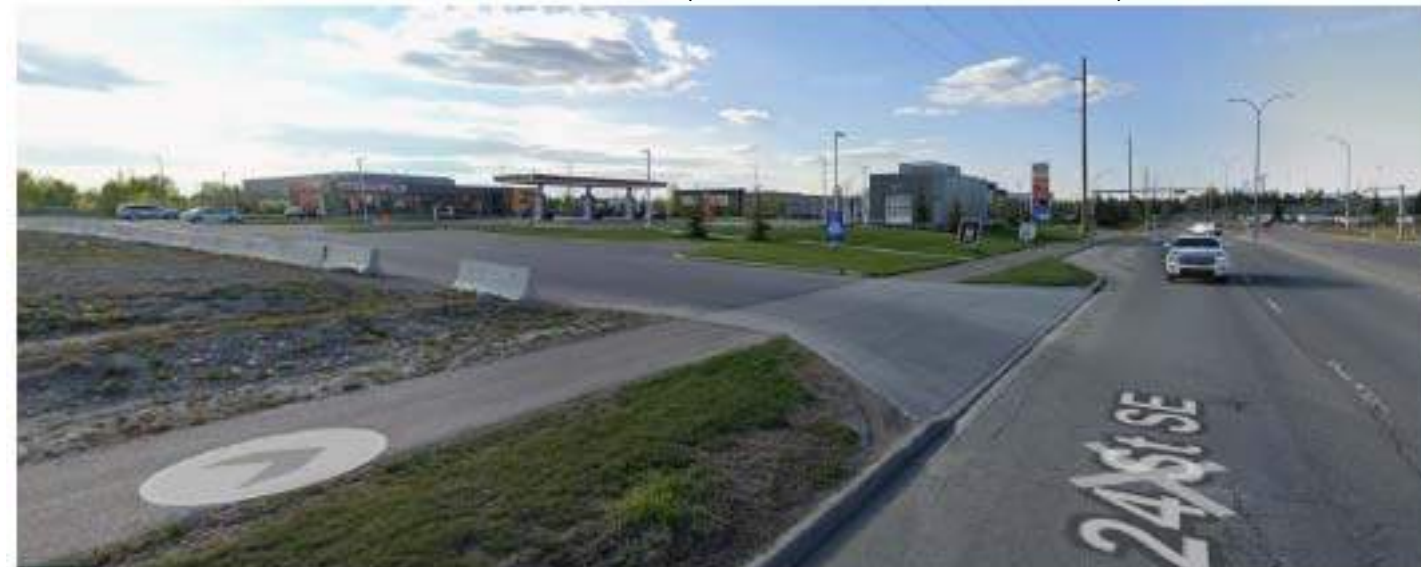
VIEW FROM NORTH EAST CORNER LOOKING NORTH WEST (ADJACENT PROPERTY TO THE NORTH)
