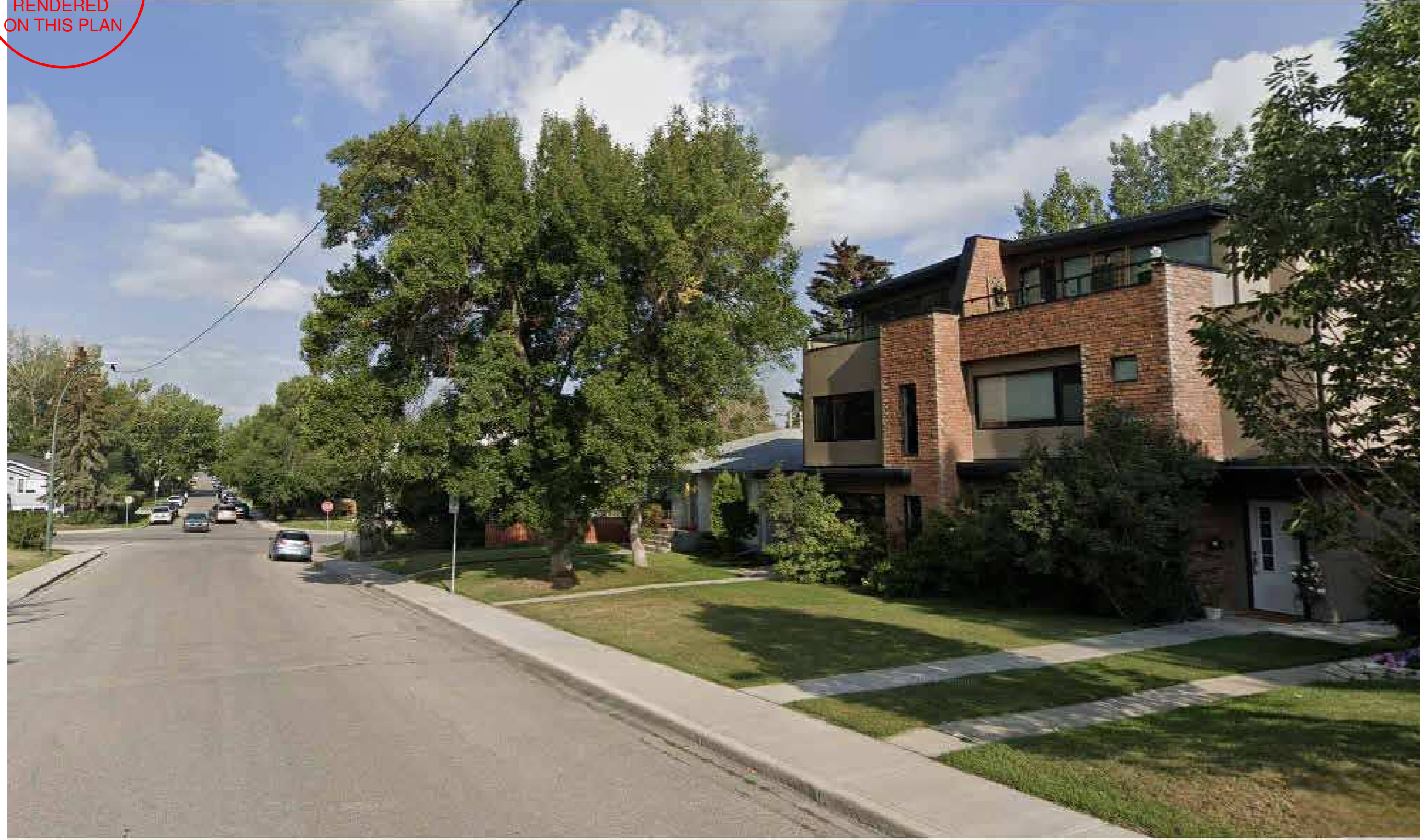
1 EAST VIEW 2136 AVE SW
