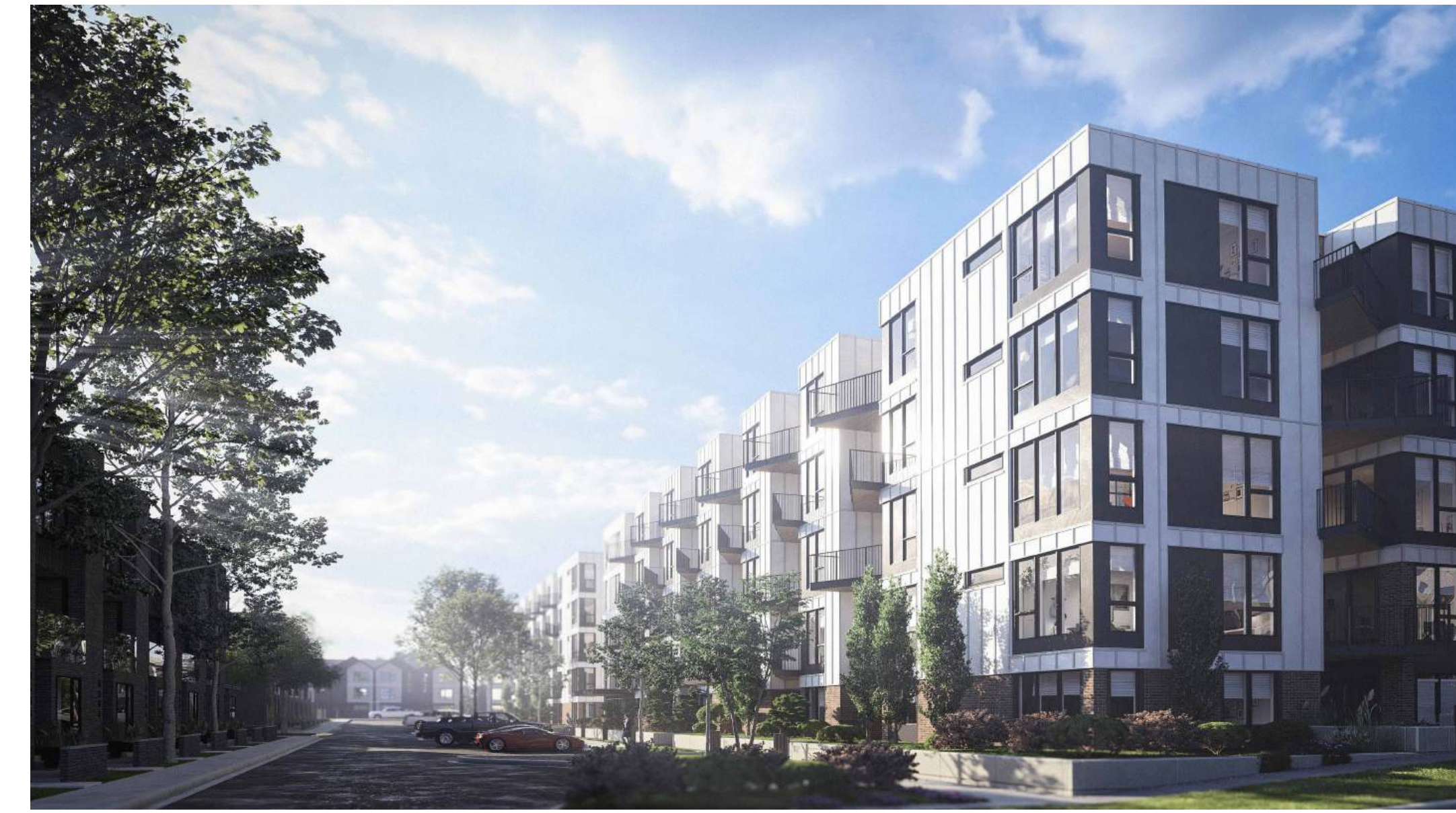
BUILDING 1 NORTHWEST CORNER
