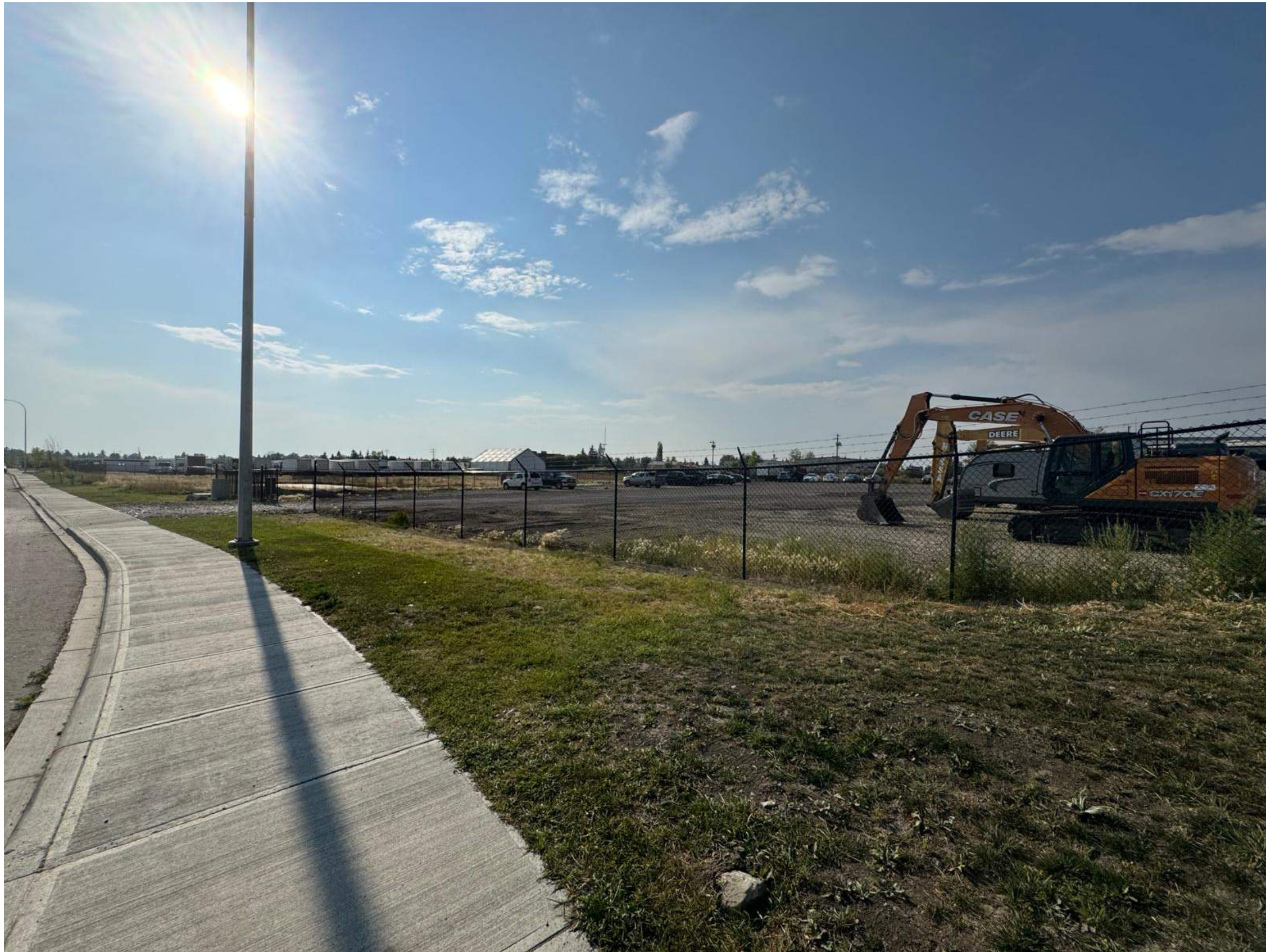
E - EAST CORNER LOT VIEW
