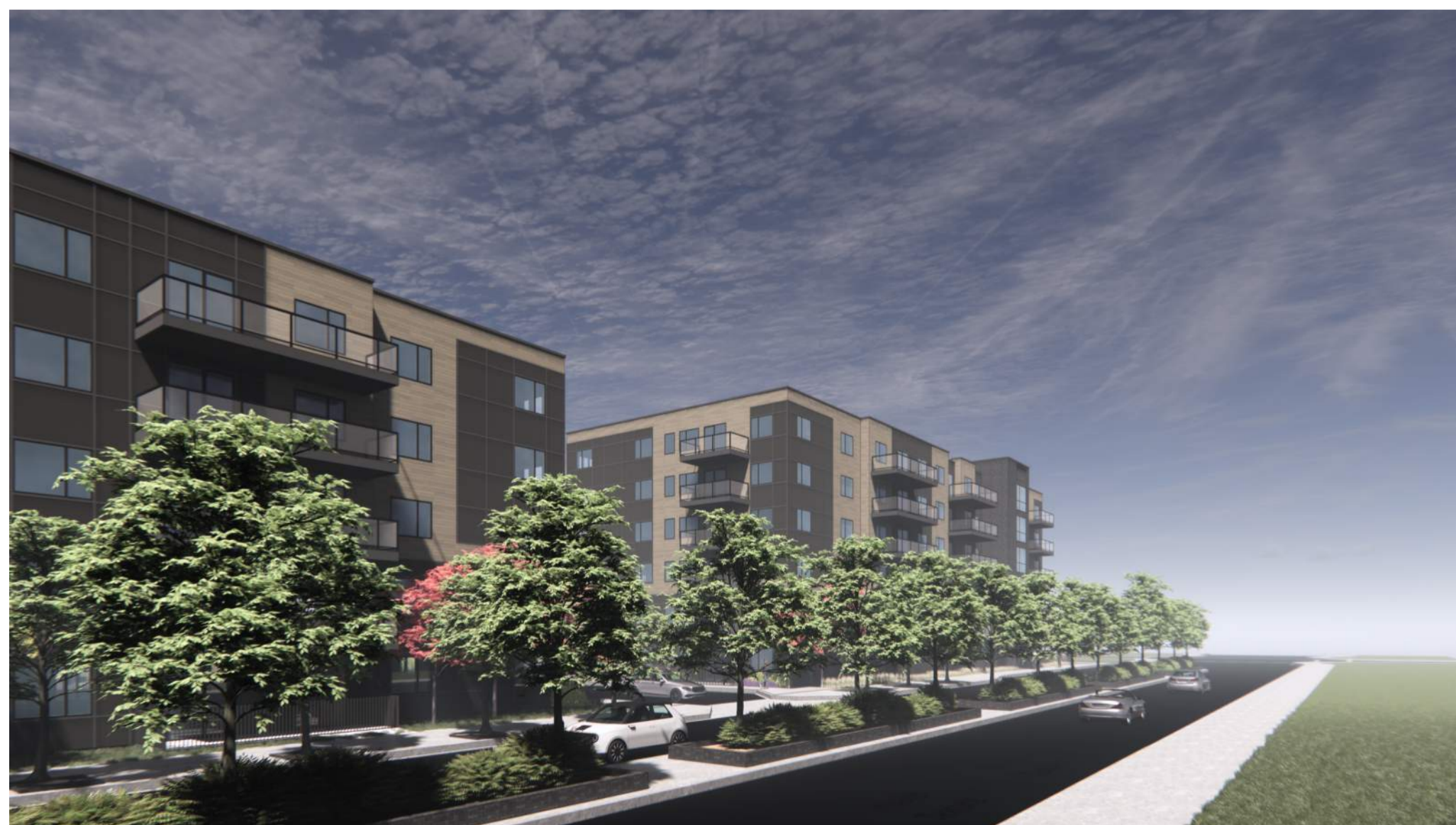
05. BUILDING A & B - VIEW FROM MARKET STREET SE
