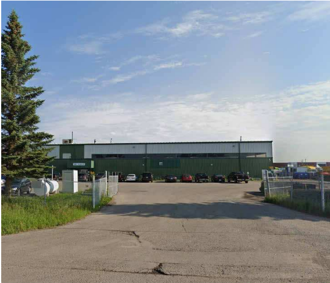
SITE PIC. #1: SOUTH ELEVATION FROM STREET
