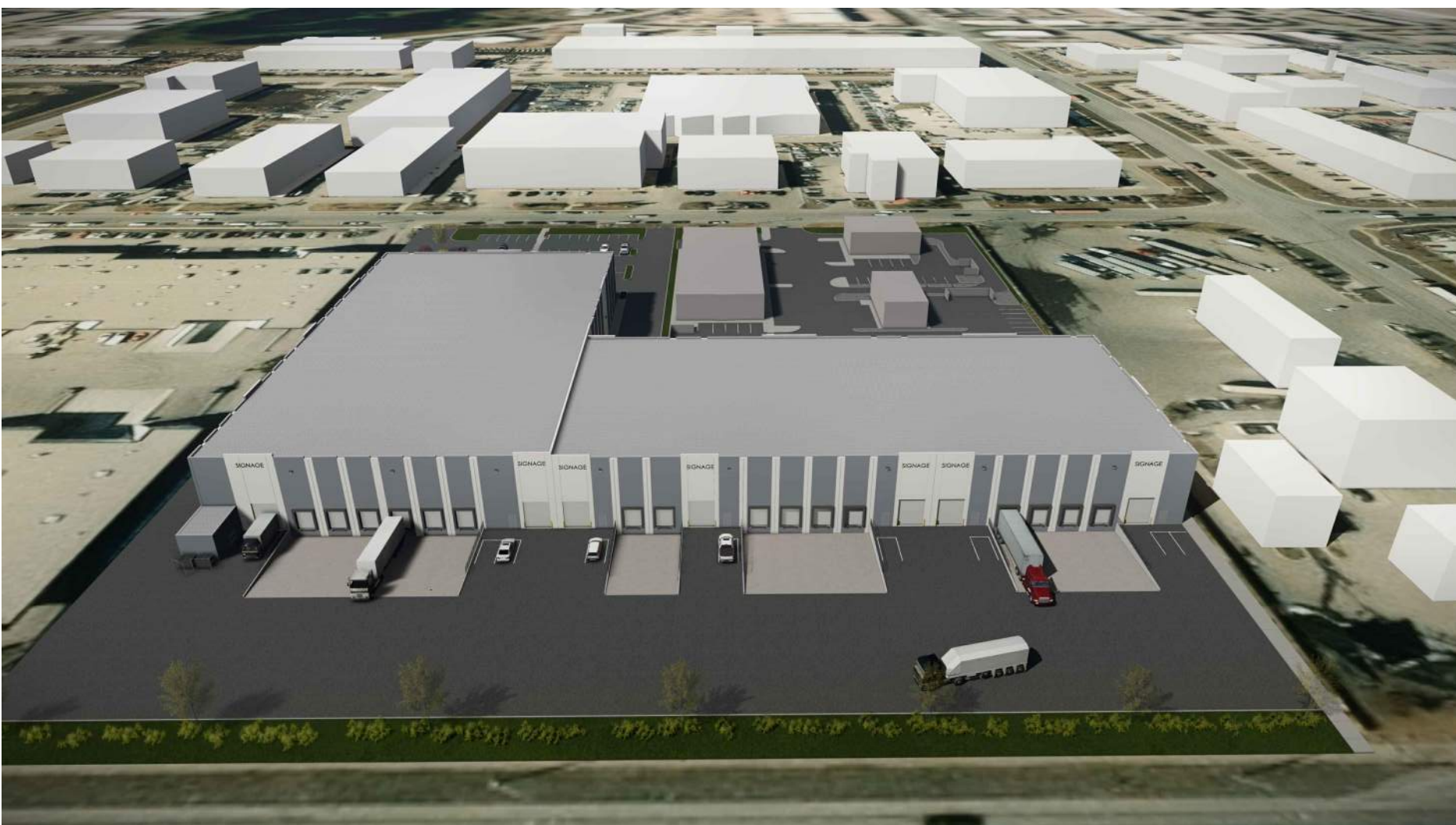
AERIAL VIEW OF LOADING
