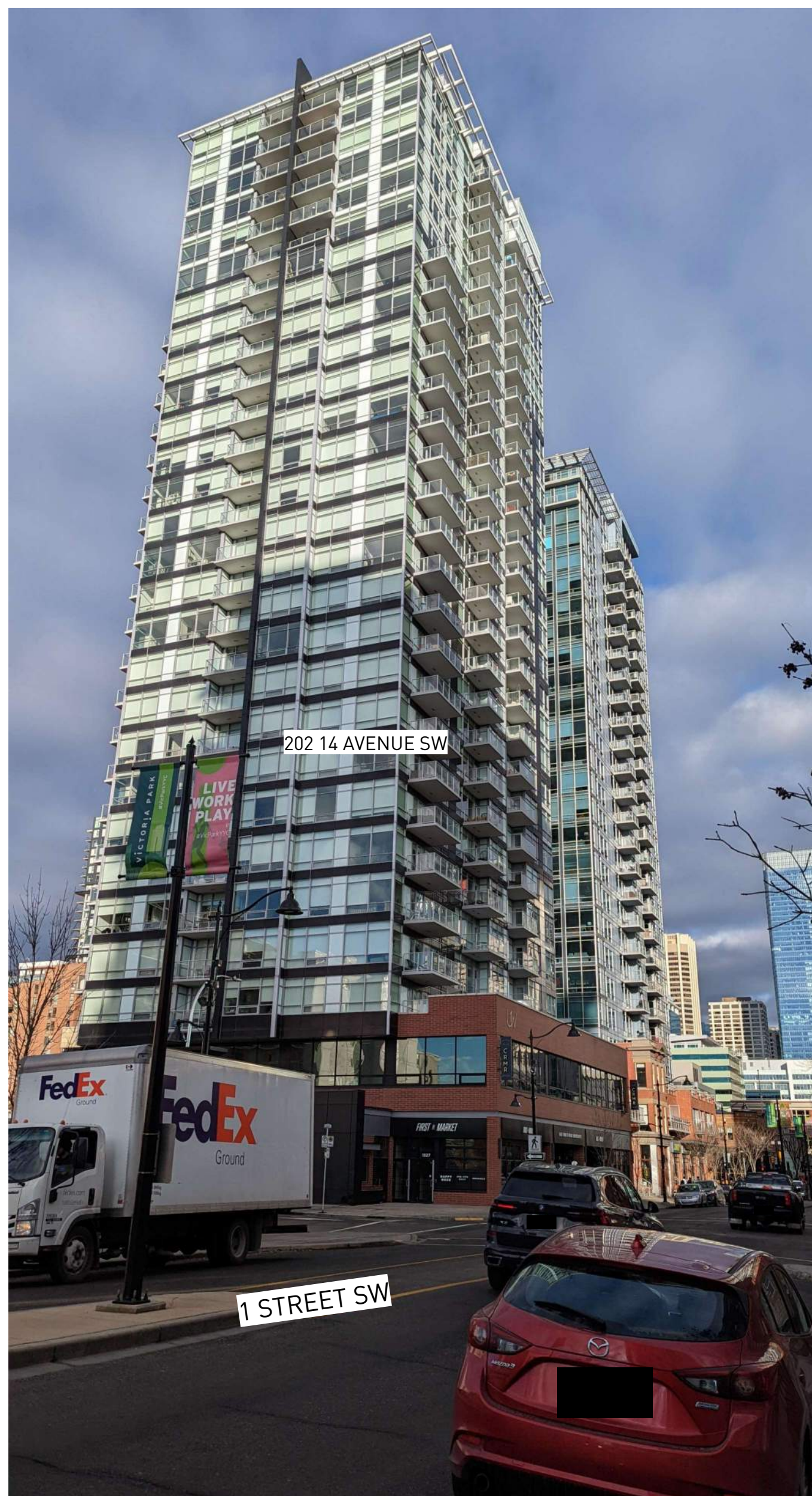
9 EXISTING SITE PHOTO FACING NORTHWEST N/A
