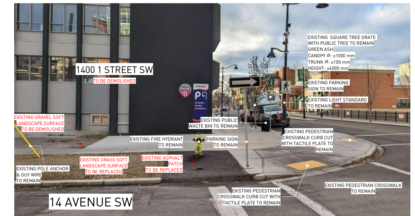
4 EXISTING SITE PHOTO FACING SOUTH N/A
