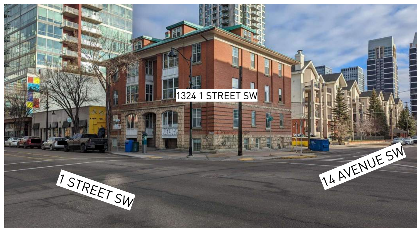
1 EXISTING SITE PHOTO FACING NORTHEAST N/A
