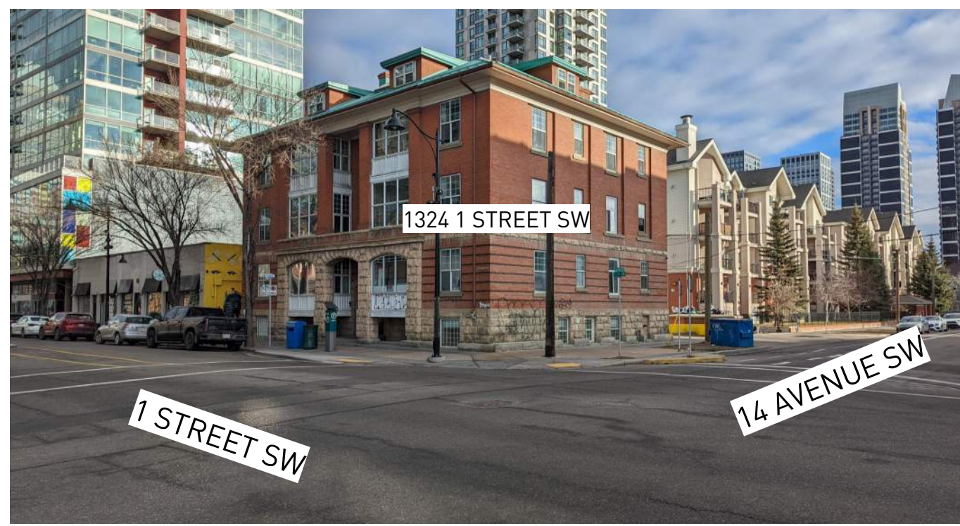
1 EXISTING SITE PHOTO FACING NORTHEAST N/A
