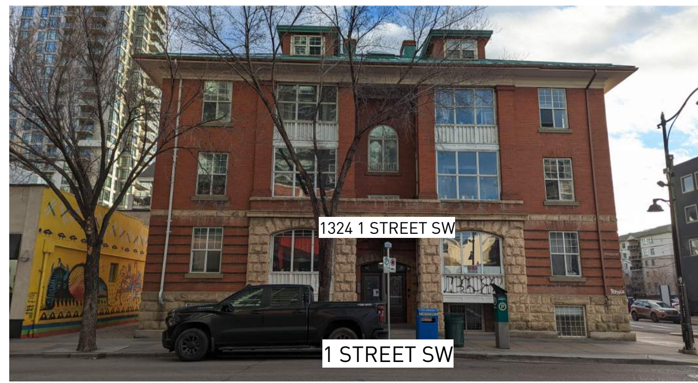
2 EXISTING SITE PHOTO FACING EAST N/A
