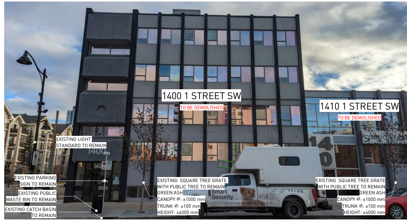
5 EXISTING SITE PHOTO FACING EAST N/A
