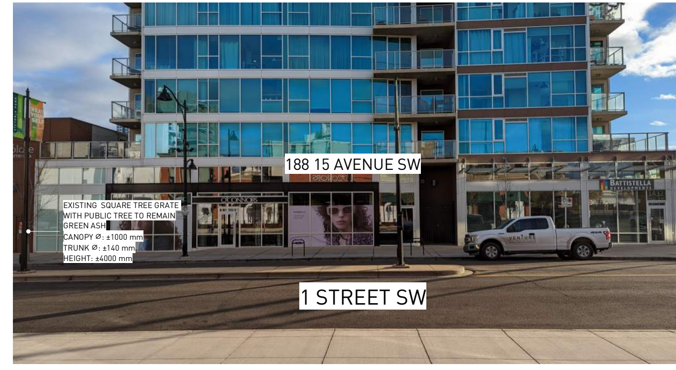
8 EXISTING SITE PHOTO FACING EAST N/A
