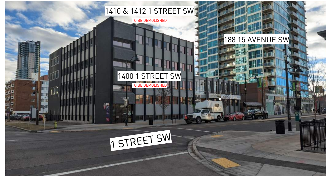
11 EXISTING SITE PHOTO FACING EAST N/A
